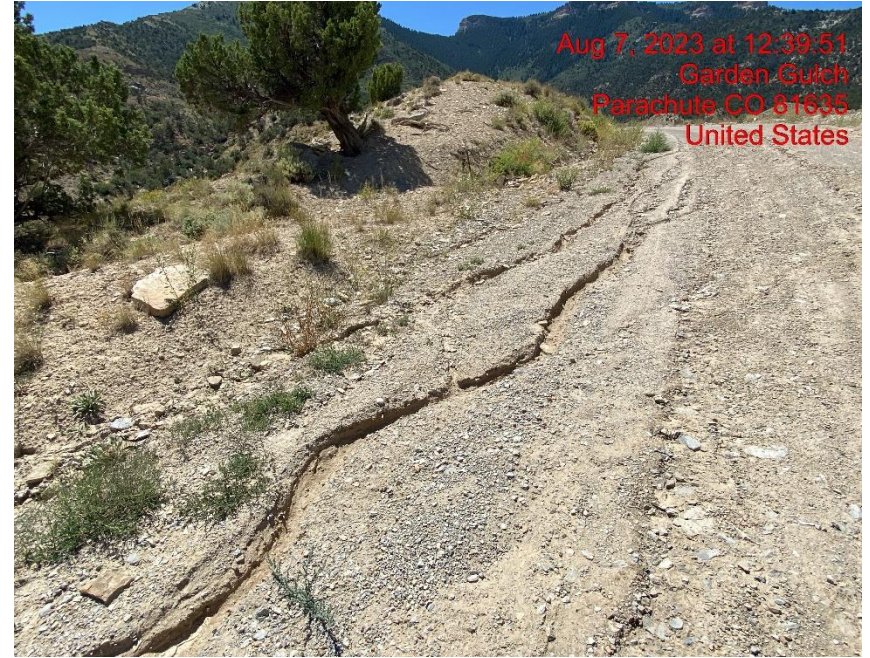
Rill Erosion Cutting Through Lease Road – Photo #05610
