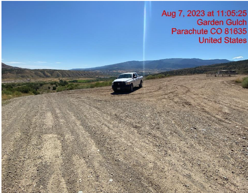
Insufficient Vehicle Tracking BMPs at Location Entrance/Exit – Photo #05540
