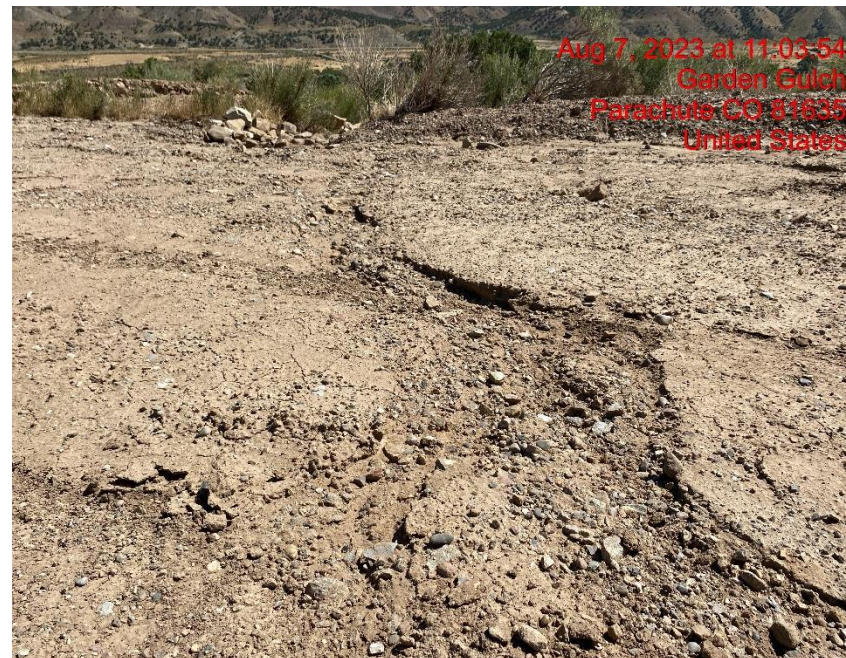
Location Lacks Stabilization – Photo #05538
