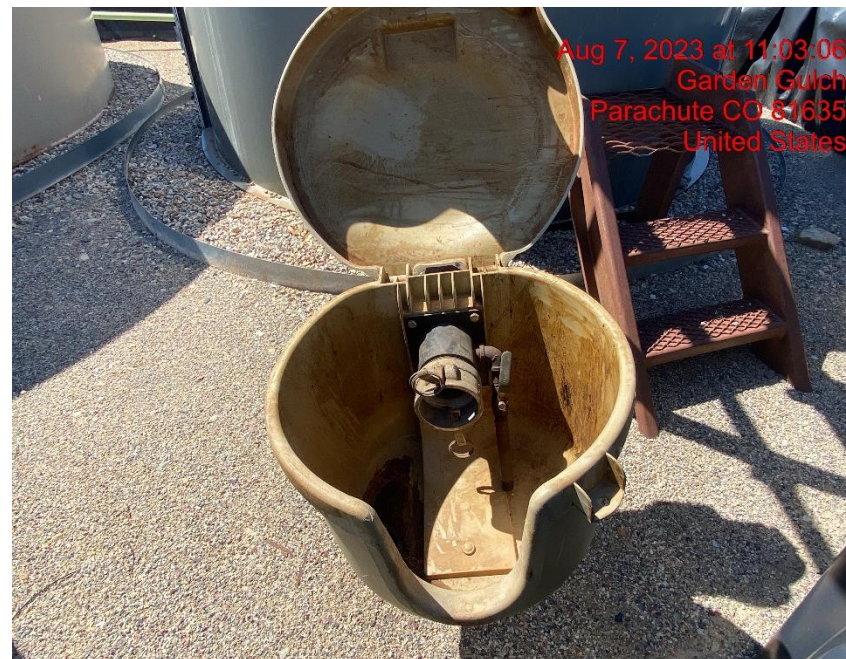
Open-Ended Load Line – Photo #05535
