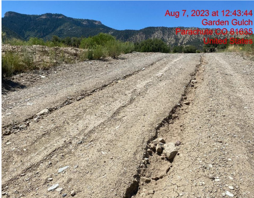
Rill Erosion Cutting Through Lease Road – Photo #05613
