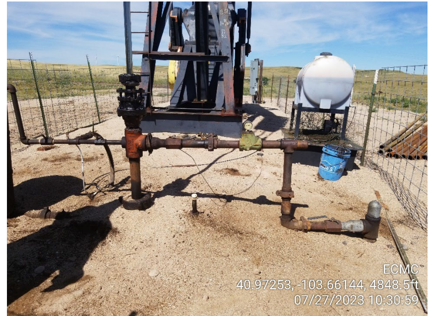
Photo 4 – Wellhead – Stained Soil
