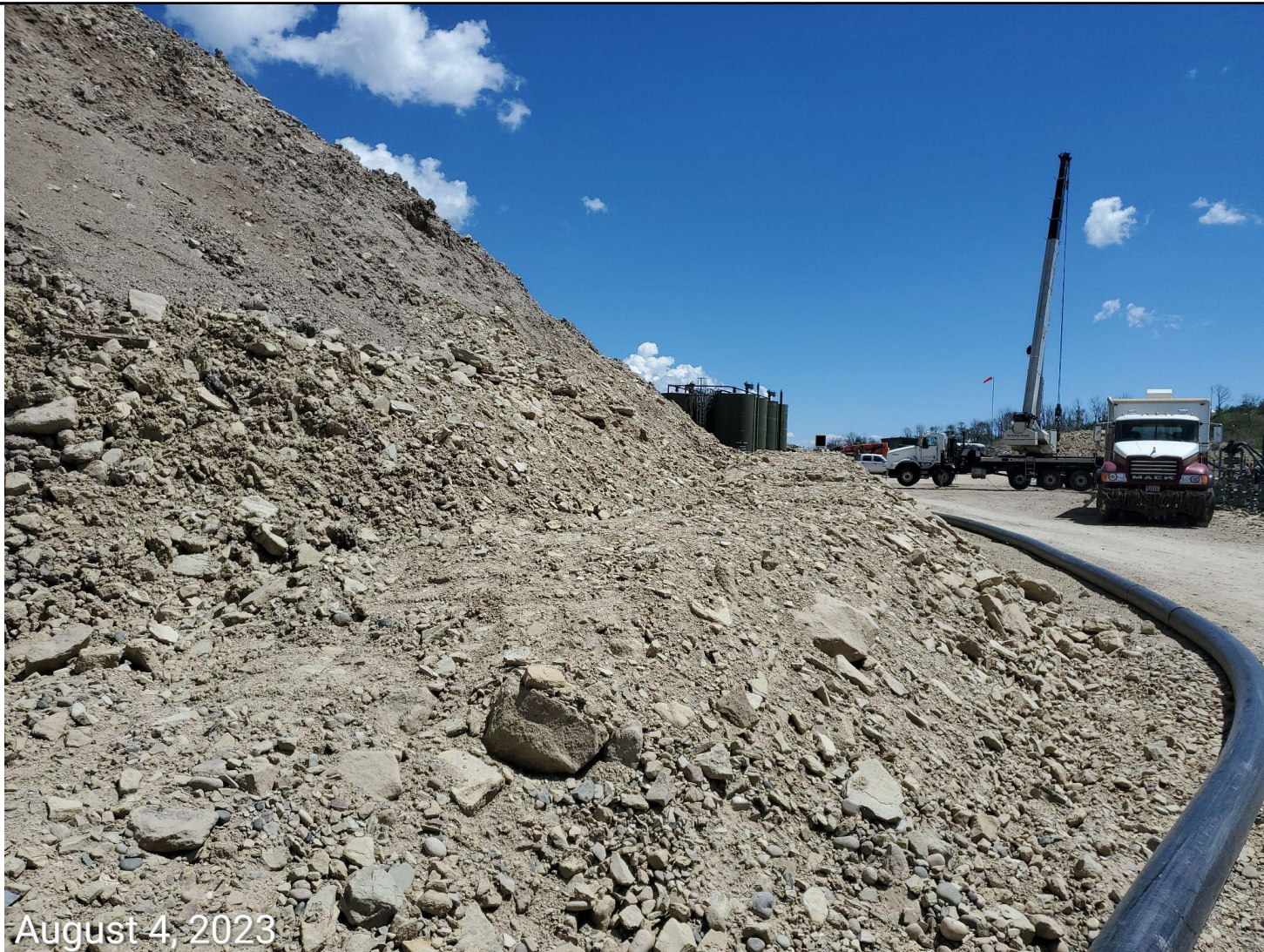
Photo 3: Photo shows Operator has installed a berm at the toe of the drill cuttings stockpiled on the north end of the Location. Berm has been installed in a manner that is inadequate to contain/prevent a spill. BMP also largely unconsolidated material.
