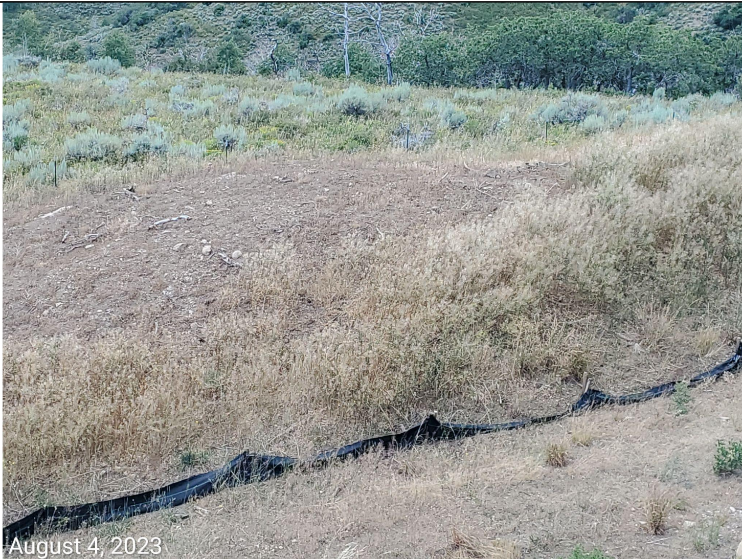
Photo 12: Photo shows topsoil stockpile on the west end of the Location. Photo shows BMPs to prevent weed establishment on the topsoil stockpiles are inadequate.
