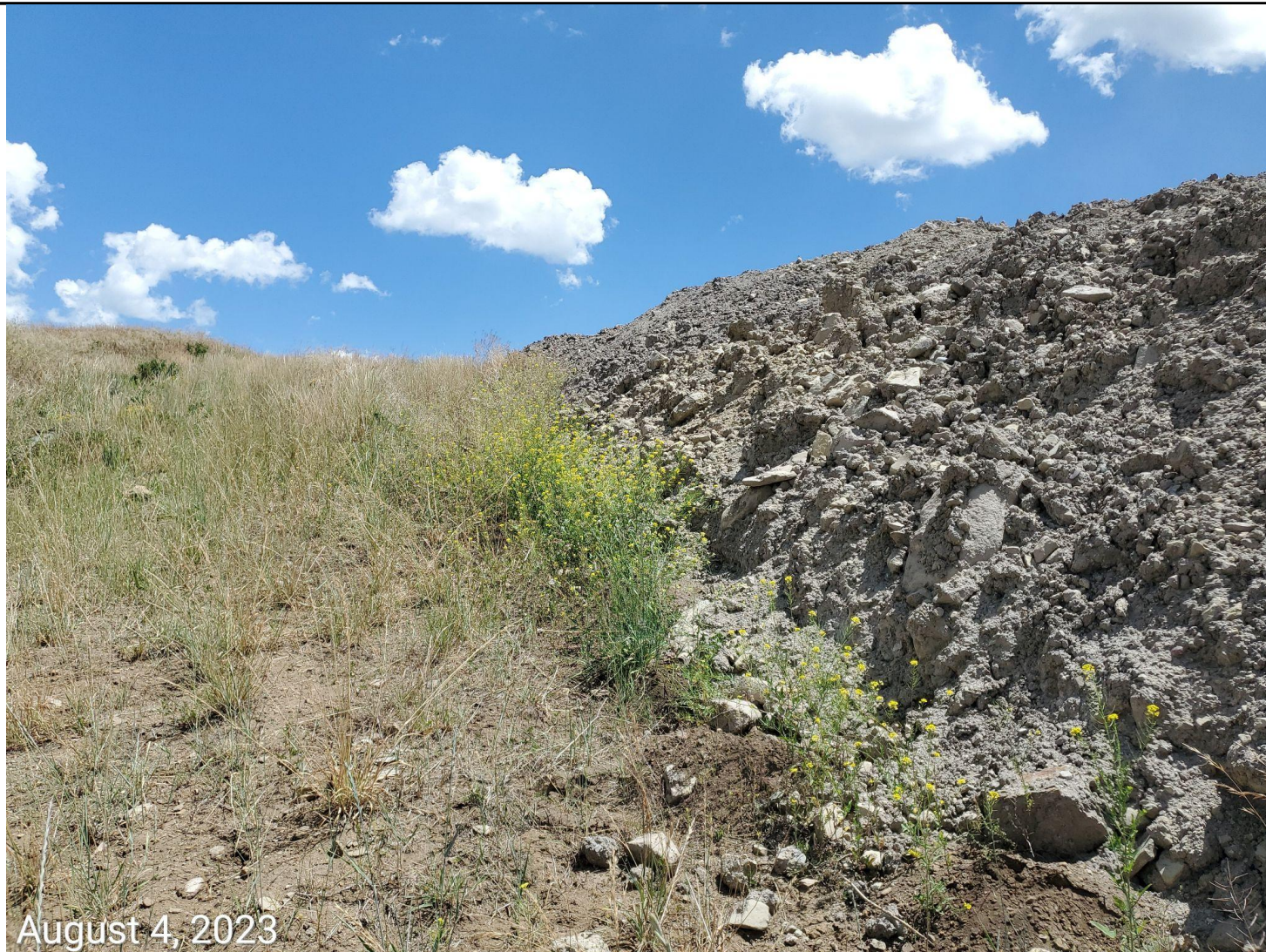
Photo 5: Photo taken from the north end of the Location, just north of the Location's cutslope. Photo shows Operator has pushed cutting material beyond the working pad surface and cutslope.
