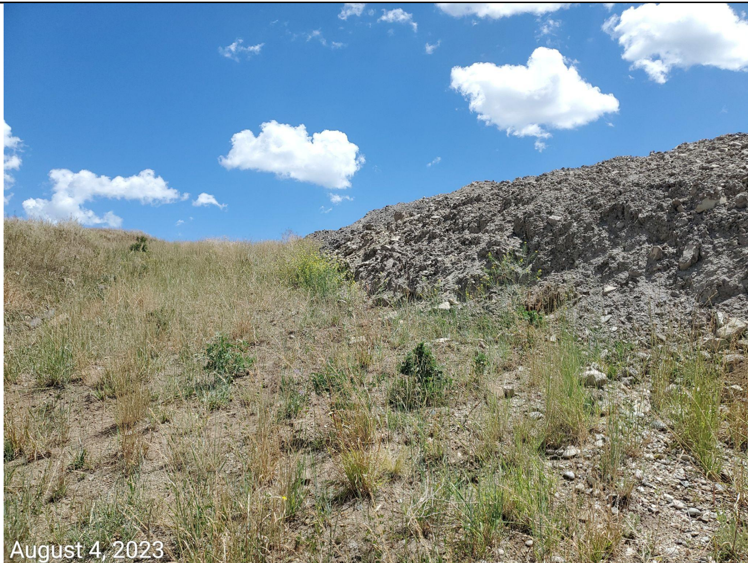
Photo 4: Photo taken from the north end of the Location, just north of the Location's cutslope. Photo shows Operator has pushed cutting material beyond the working pad surface and cutslope.
