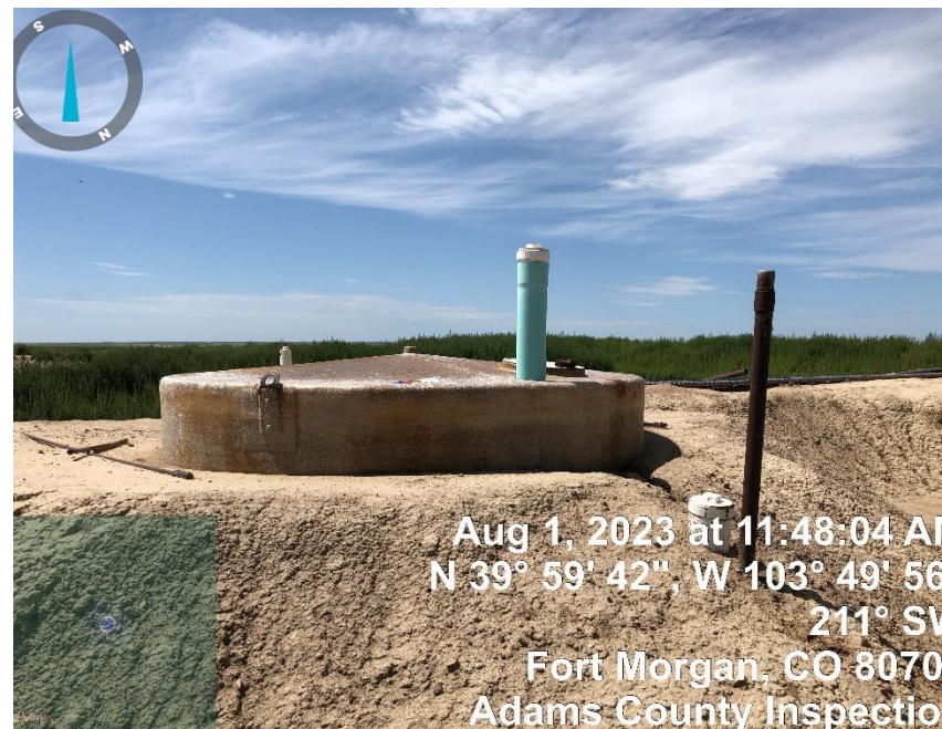
Photo#4 Produced Water Tank (NO BBL markings and identification labels).
