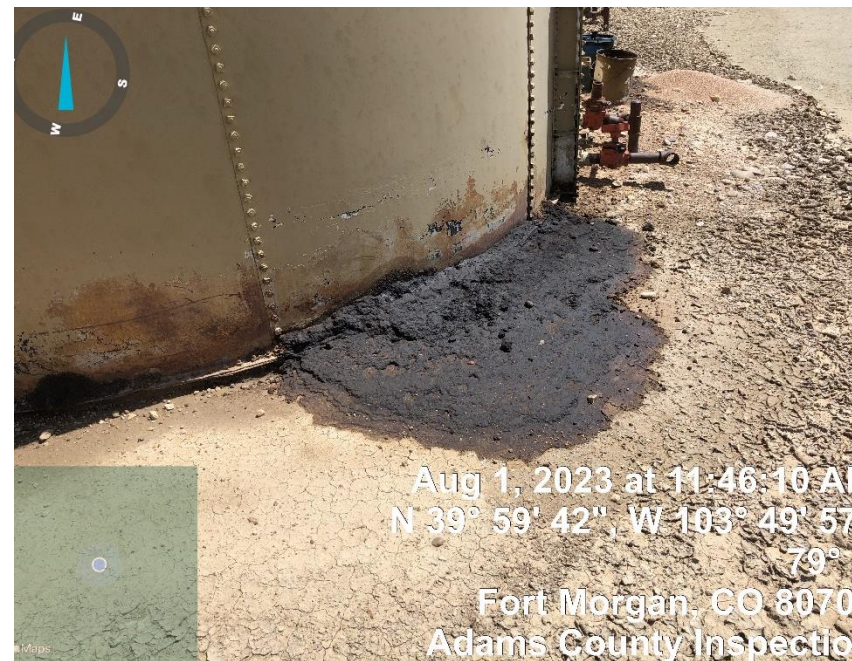
Photo#2 Stained Soil behind SW Production Tank
