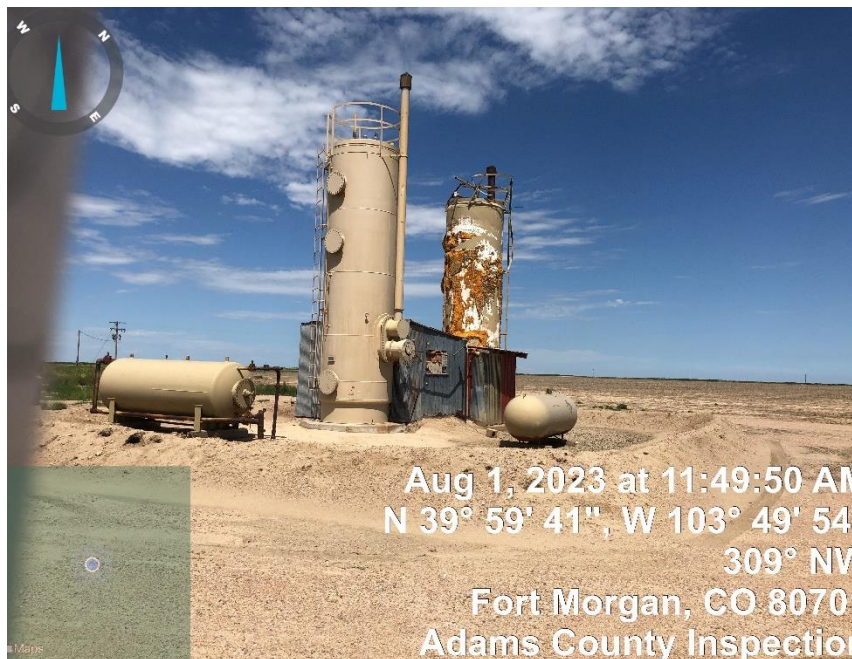
Photo#9 (2) Vertical Separators/Propane Tank/Buffer Tank
