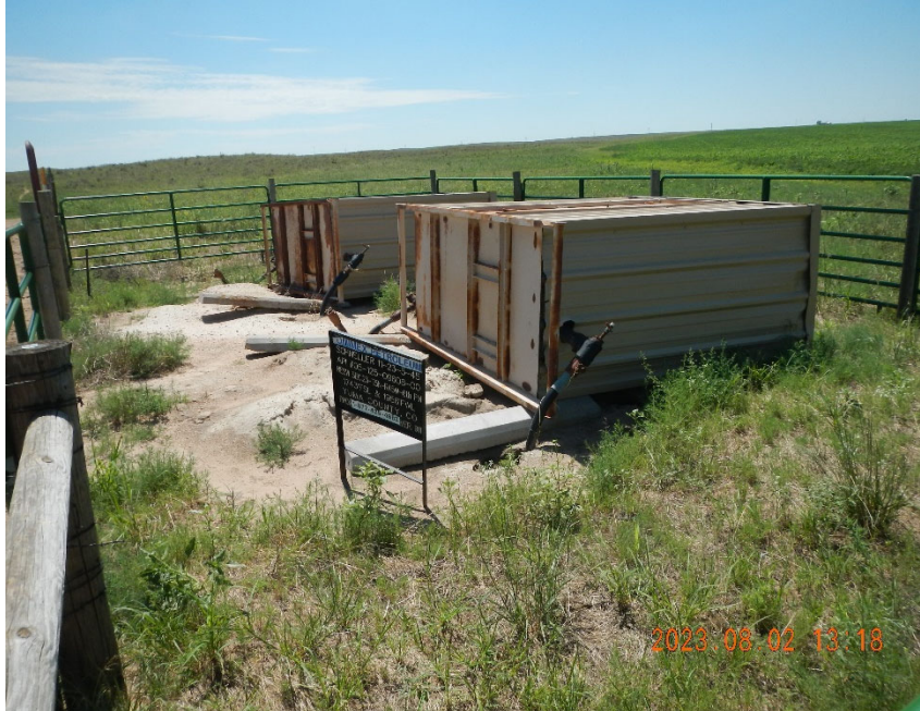
7. Additional view of blown over Meter Shed.
