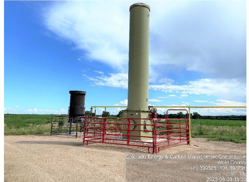
Photo #4 Lohr 32-13 Battery site Inactive | Shut-down ECD(s)
