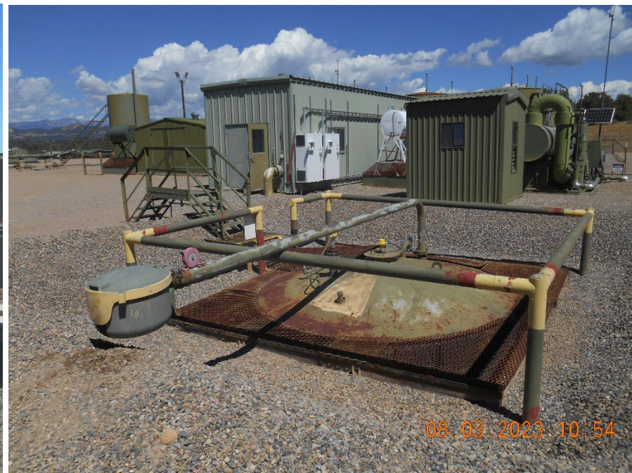
Pump housing and blowdown tank
