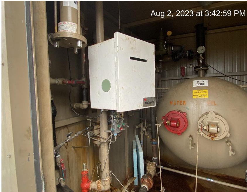
No visible display of gas calibration
