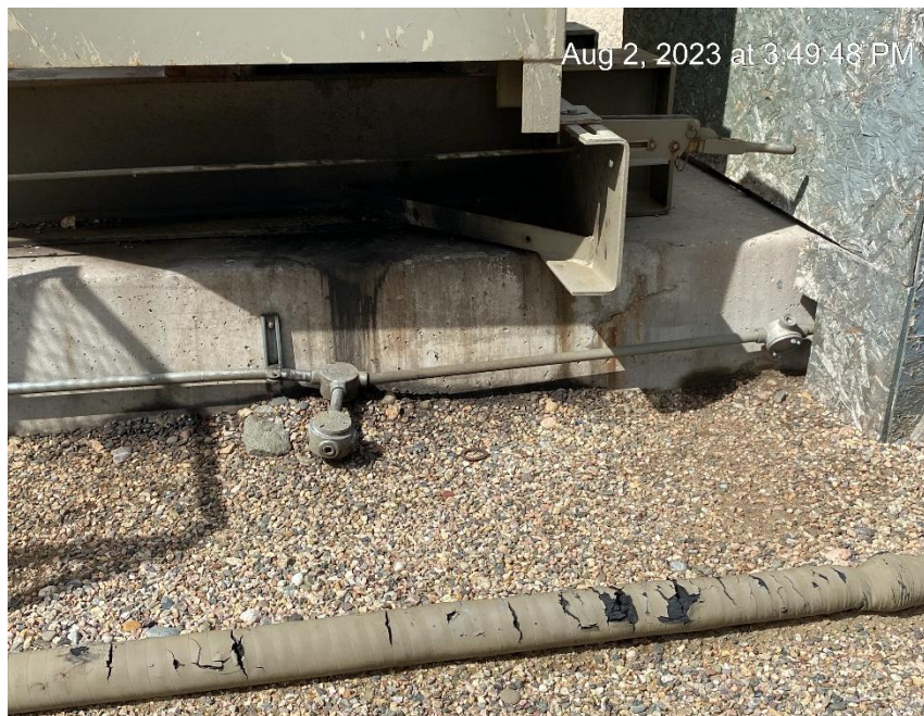
Engine leakage. Stained soil.
