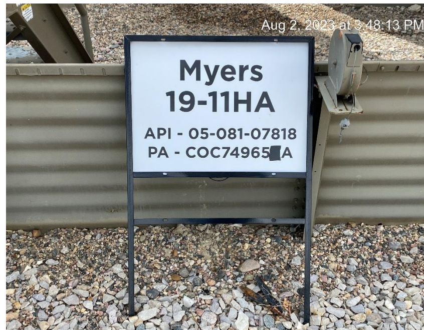
Tank battery sign missing required information
