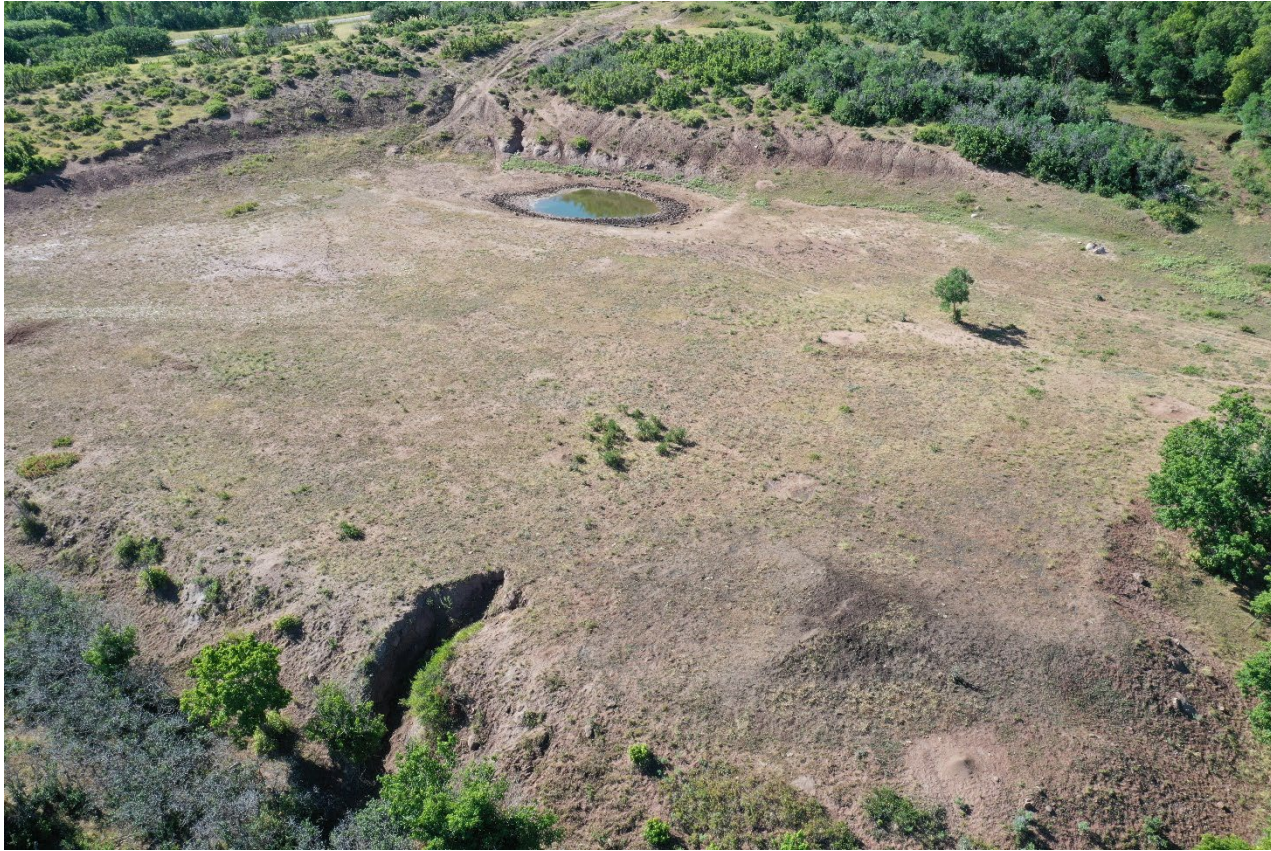
Photo 5. Facing south at the location. There is a large erosion gully along the fill slope shown at red arrow..
