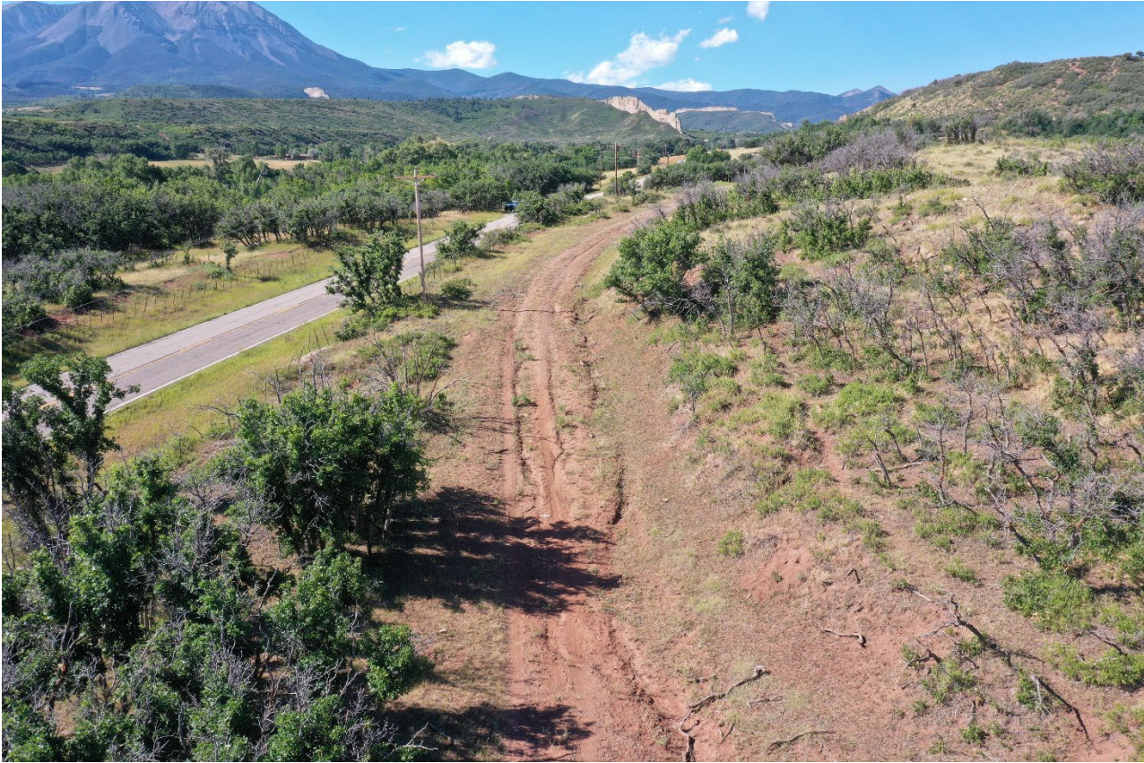
Photo 2. Facing southwest along the access road. There is signs or erosion along the road.
