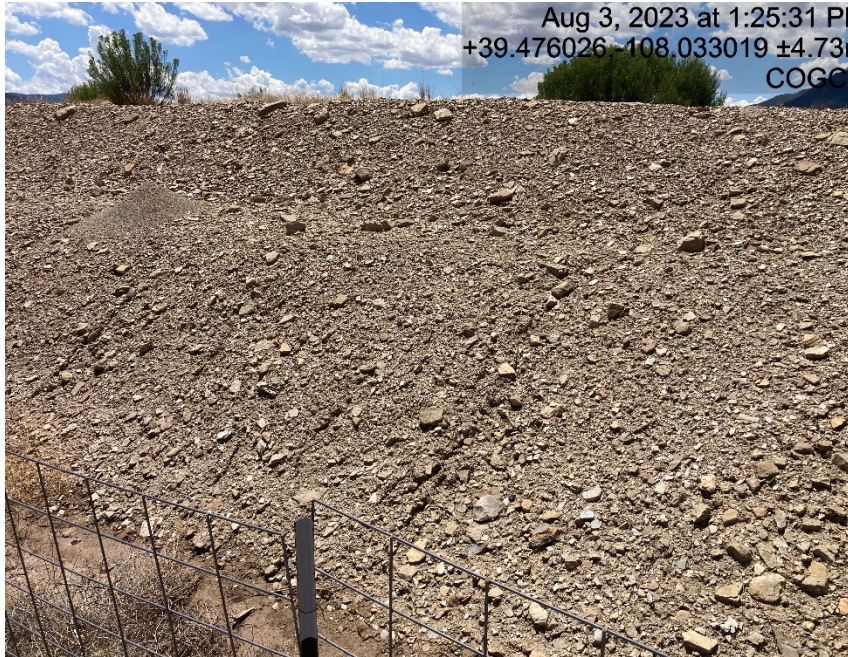
Cut slope lacks stabilization
