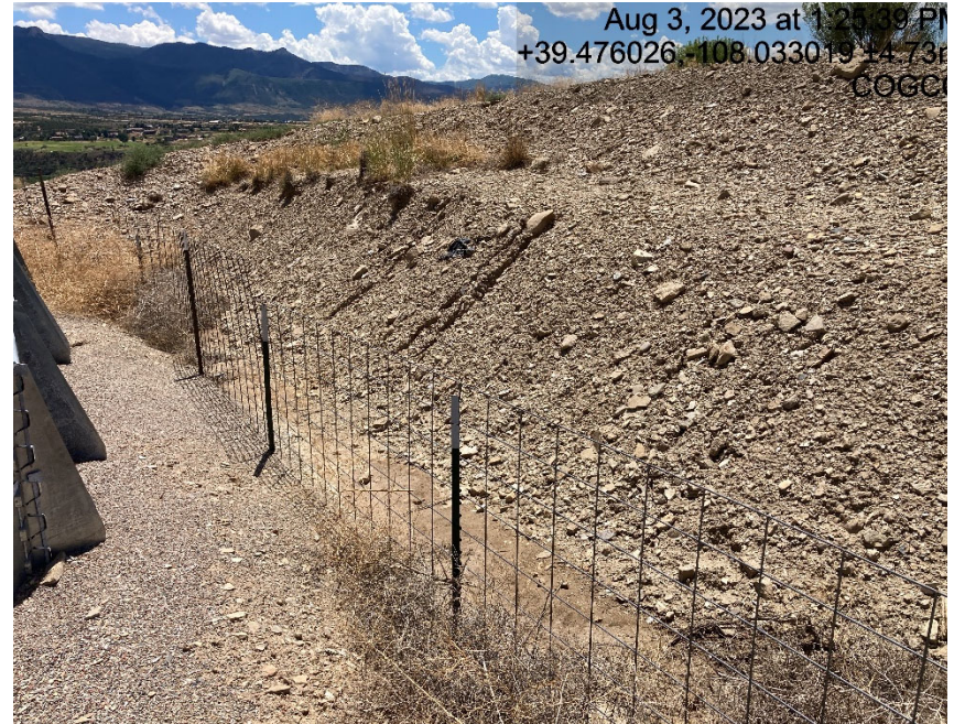
Cut slope lacks stabilization
