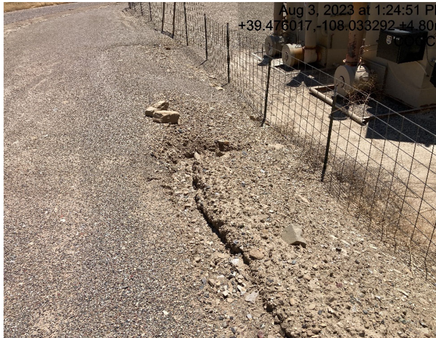
Erosion on cut slope causing run on
