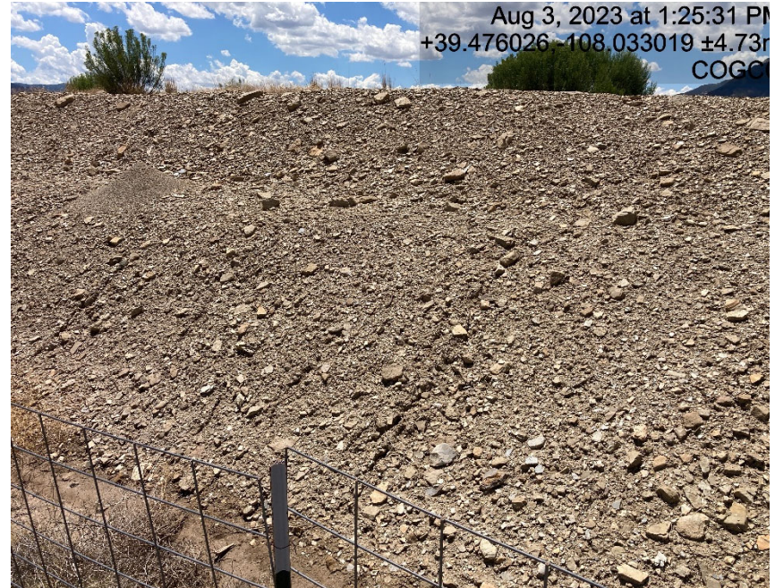
Cut slope lacks stabilization
