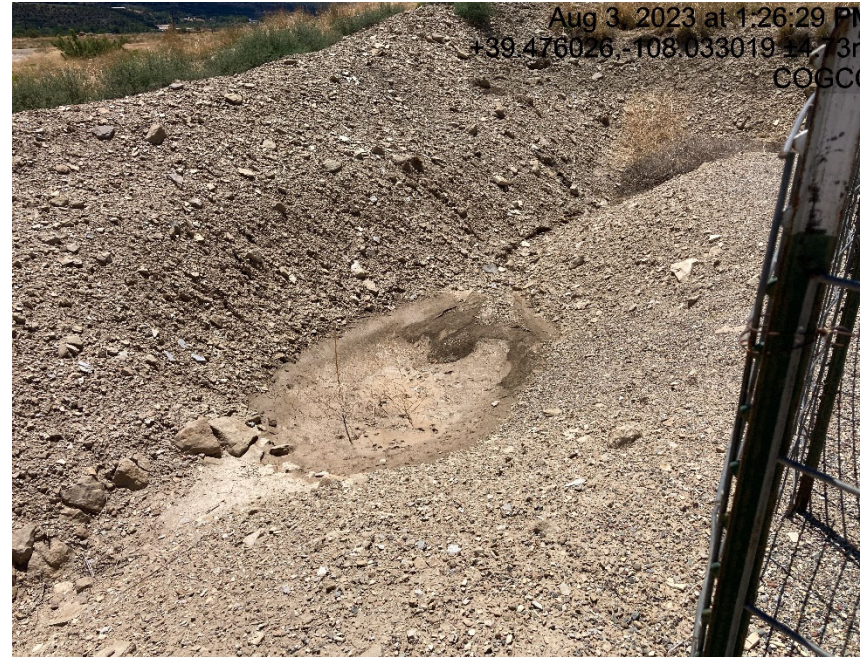
Cut slope lacks stabilization
