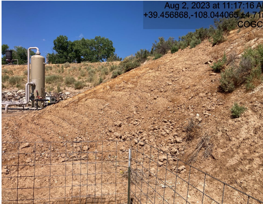
Fill slope has been hydroseeded
