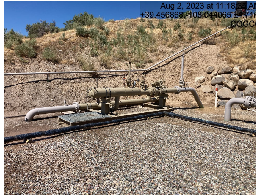
Cut slope behind pig station lacks stabilization
