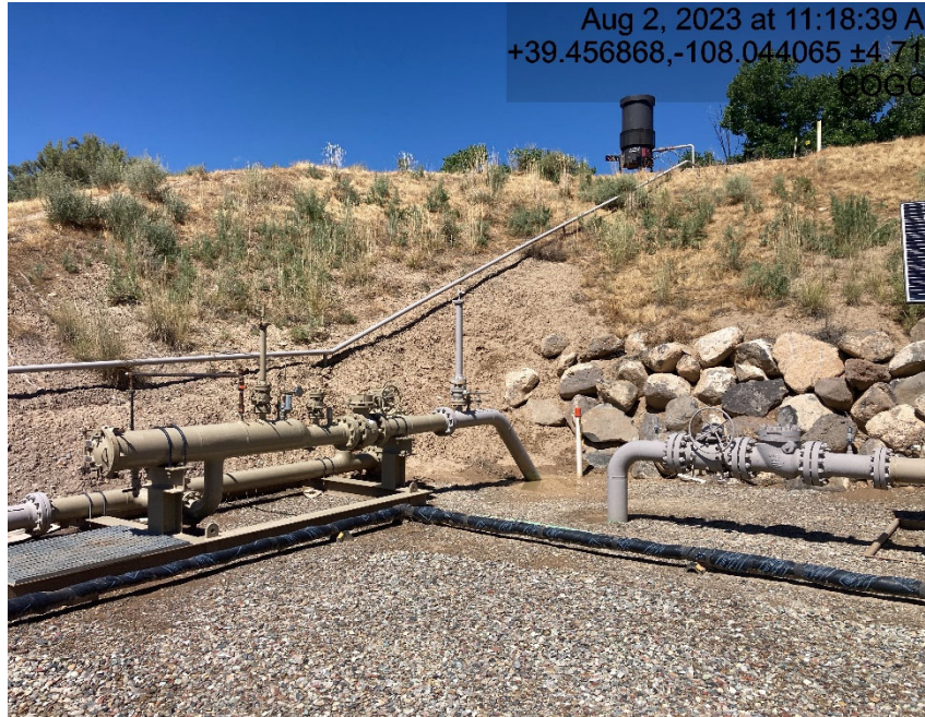
Cut slope behind pig station lacks stabilization
