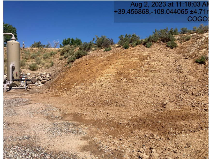
Fill slope has been hydroseeded
