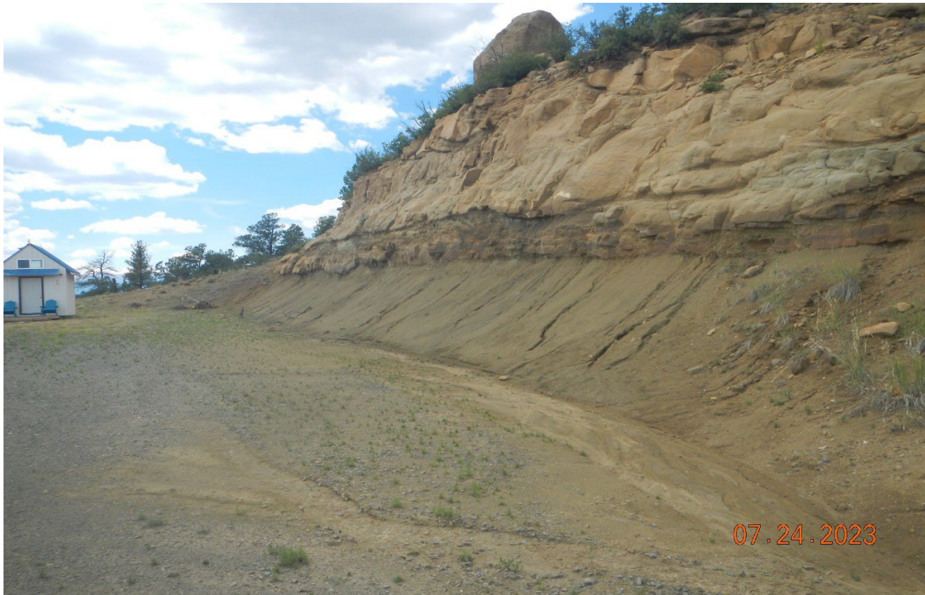
Photo 11. Facing northwest toward the cut slope. There appears to be some unstable rock along the cutslope which may fall onto the wellpad. BMP's will need to be installed for stabilization of the cut slope and rock/sediment movement.
