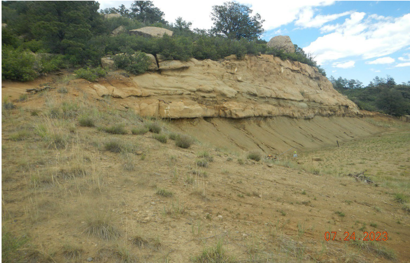
Photo 10. Facing northeast toward the cut slope. There are areas of bare soil and rill erosion.
