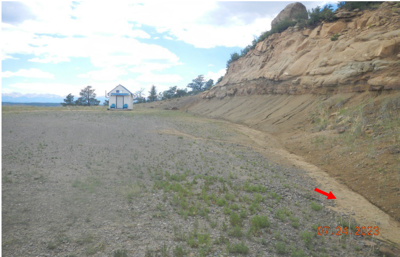
Photo 4. Facing west toward the location. There is sediment deposition shown at red arrow. BMP's will need to be installed to prevent sediment migration offsite. The landowner has placed a shed on the location.
