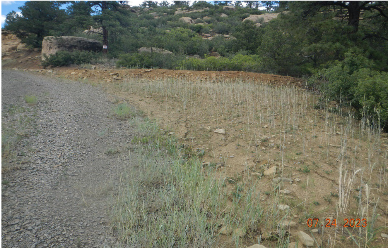
Photo 3. Facing northwest near the location. A diversion berm was placed to divert stormwater off the road. This area was reseeded but has not yet established sufficient vegetation cover for stabilization.
