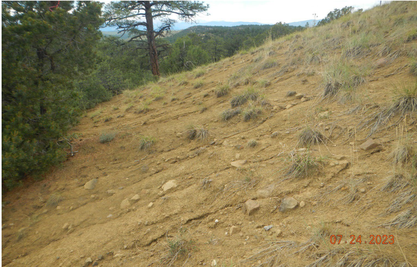
Photo 8. Facing northwest at the bottom of the fill slope. There are areas at the base of the fill slope that are not stabilized and have rill erosion occurring.
