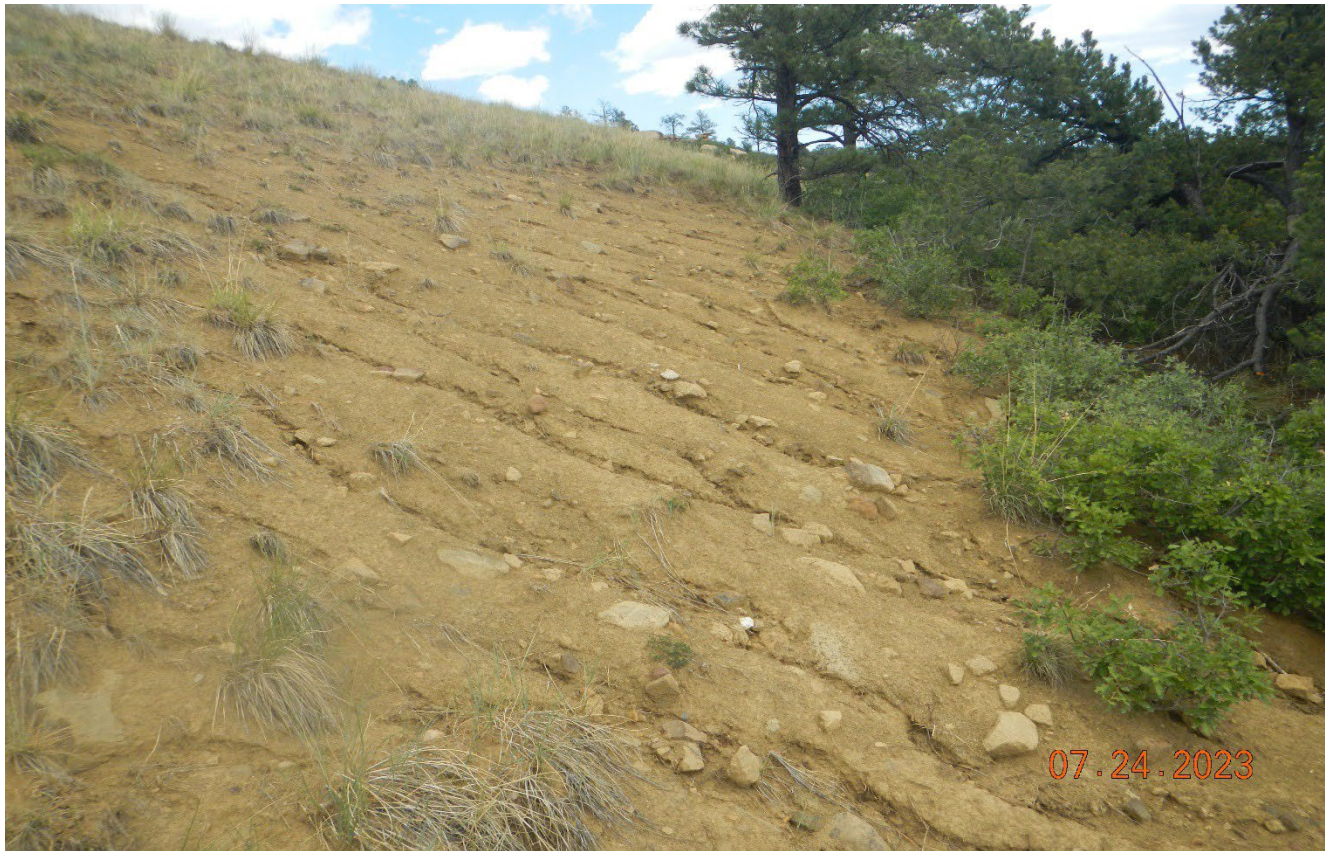
Photo 7. Facing northeast at the bottom of the fill slope. There are areas at the base of the fill slope that are not stabilized and have rill erosion occurring.
