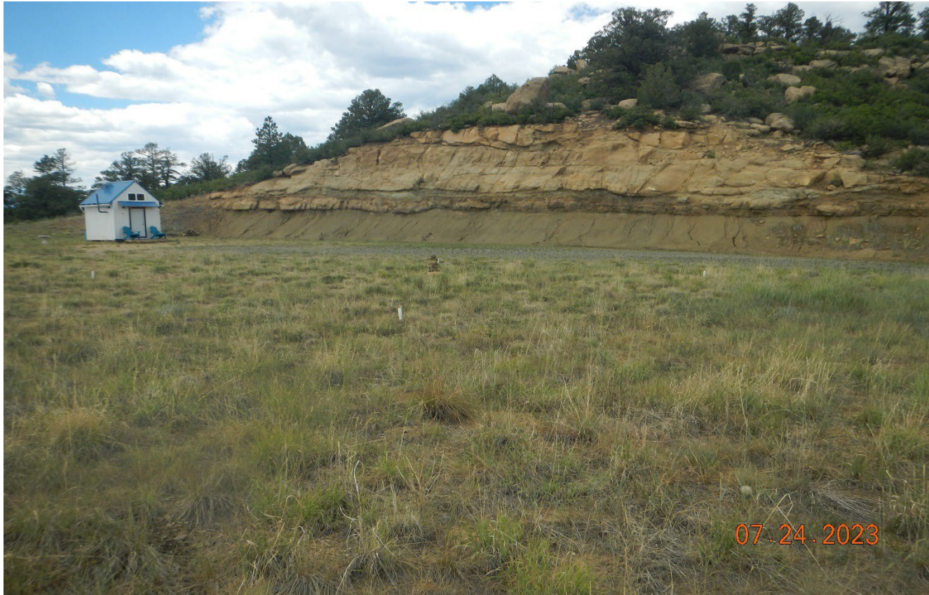
Photo 5. Facing northwest at the location. The well has been cut and capped below grade and there is no above ground well marker. All oil and gas equipment has been removed. The landowner has placed a shed on the location.
