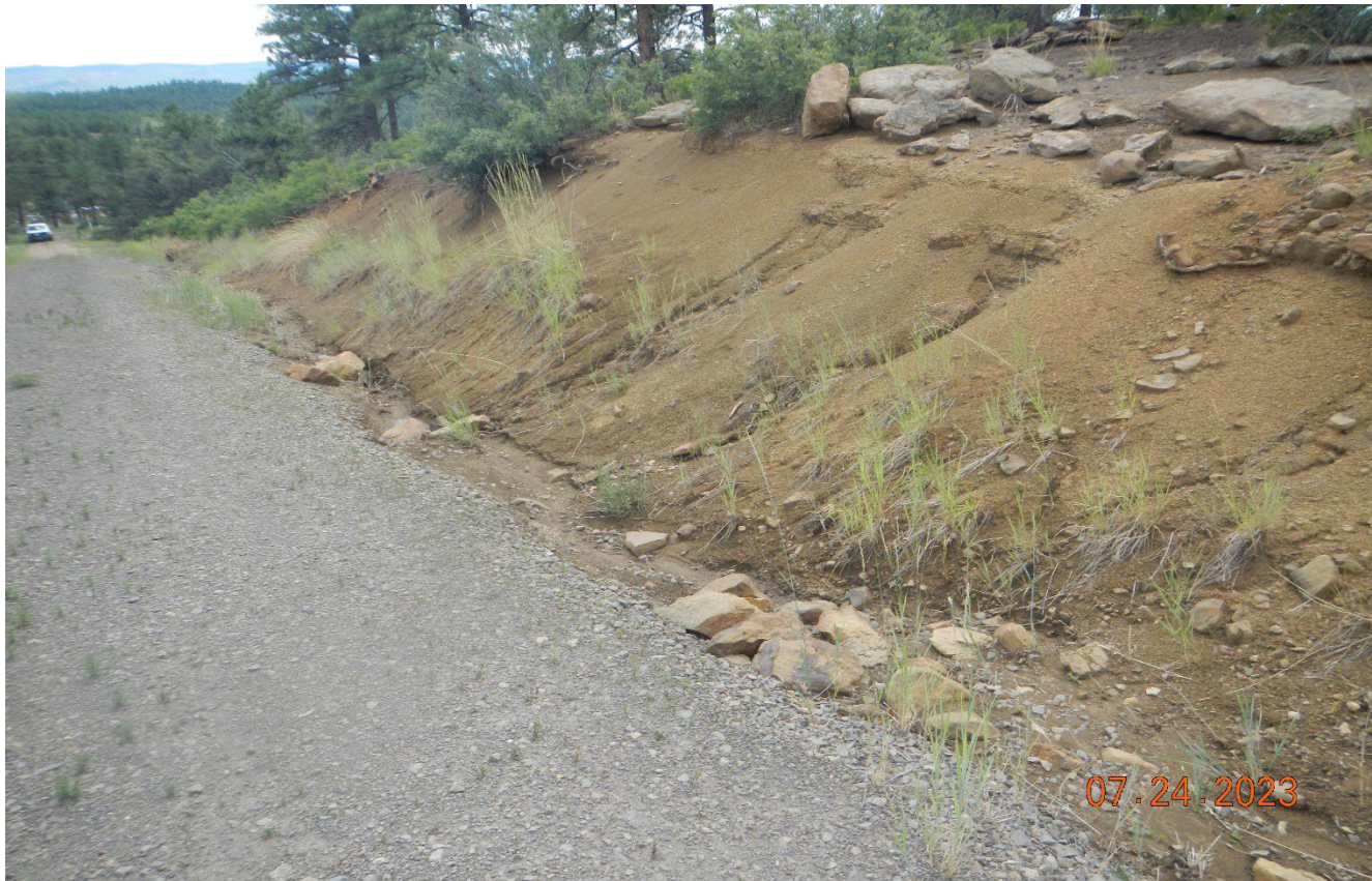
Photo 2. Facing southwest along the roadside. The rock check dams are not functioning or maintained and the roadside is not stabilized. Bare soil and rill erosion evident.
