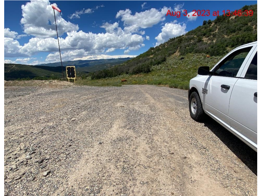
Insufficient Vehicle Tracking BMPs at Location Entrance/Exit – Photo #05458
