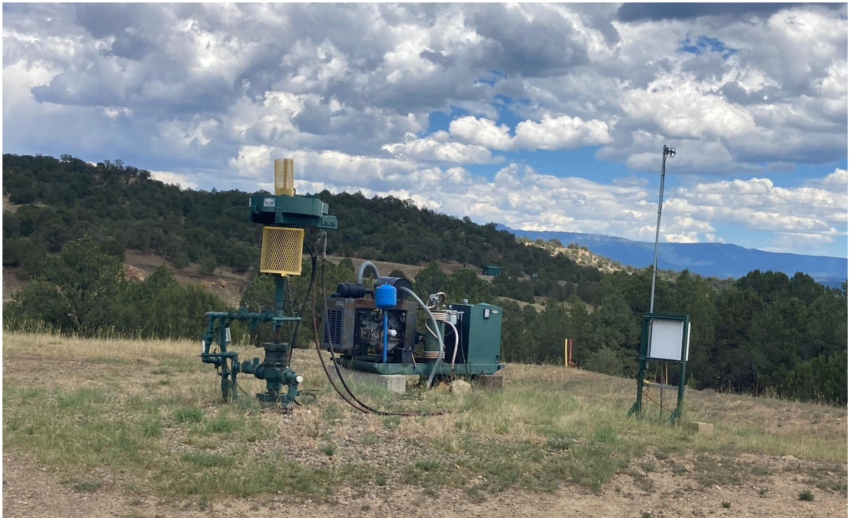
PHOTO 3: WELLHEAD AND EQUIPMENT
