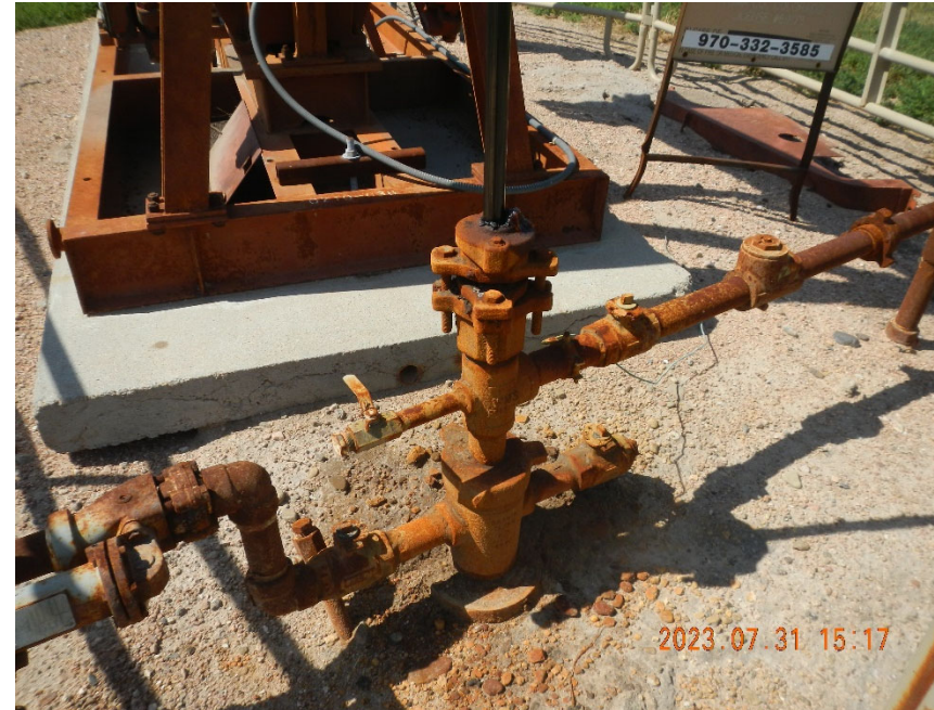
2. View of Wellhead. Note stained soil.
