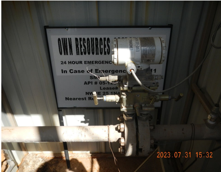
5. Digital Gas Meter inside Meter Shed.
