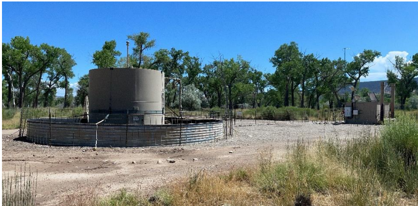
South West corner of location.
