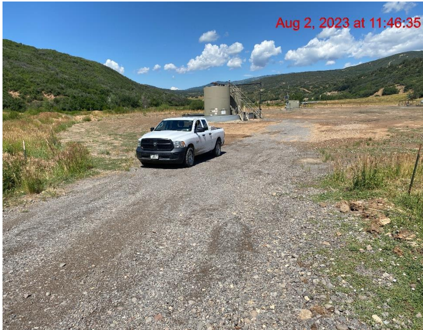
Insufficient Vehicle Tracking BMPs at Location Entrance/Exit – Photo #05375
