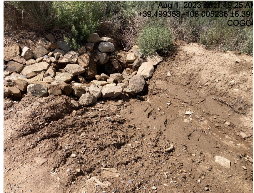
Sediment trap is failing and under mined
