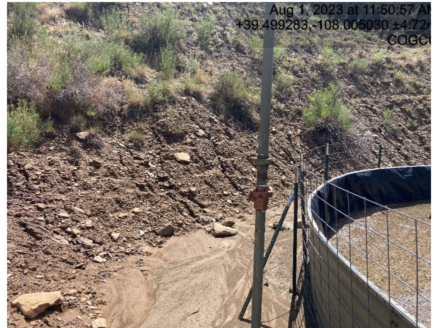
Lack of stabilization on cut slope and riling
