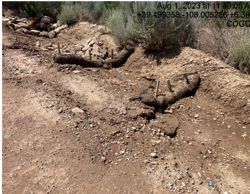
Waddle is failing
