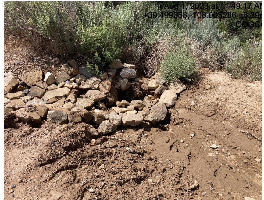
Sediment trap is failing and under mined
