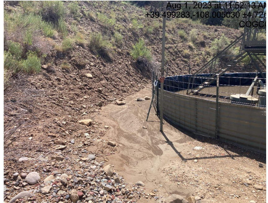
Lack of stabilization on cut slope
