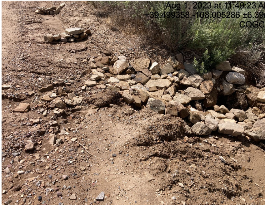
Sediment trap is failing and under mined
