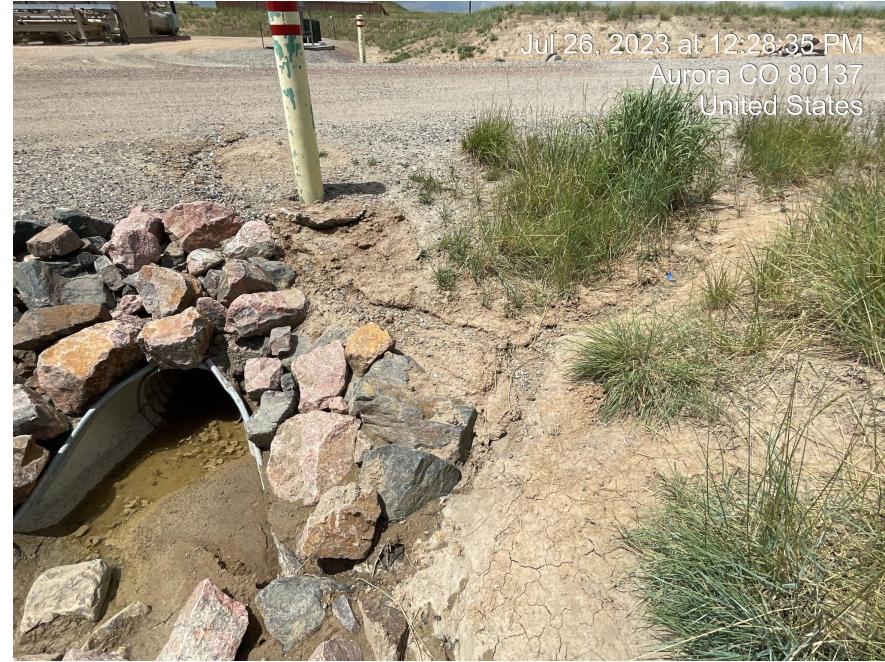
Photo 4. Stormwater erosion above culvert from access road.
