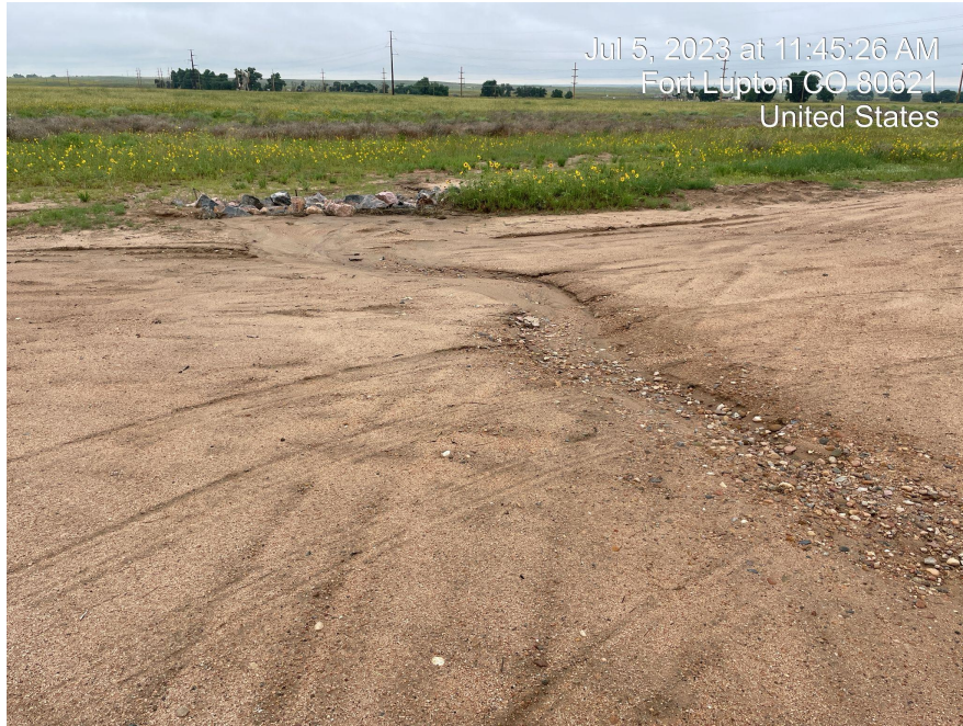
Photo 3. Photo of Stormwater erosion on site.
