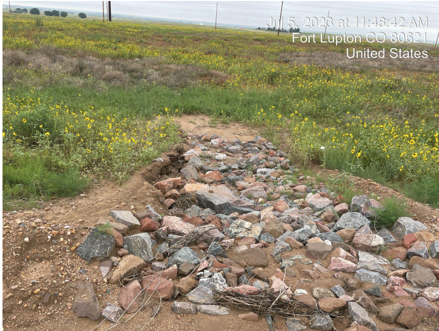
Photo 9. Photo of rock run down filled with sediment.
