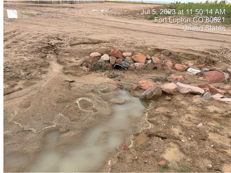
Photo 10. Photo of buried culvert at pad entrance of pad
