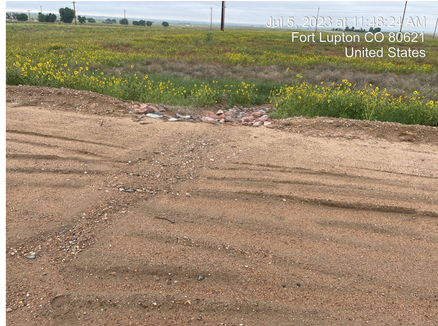
Photo 8. Photo of stormwater erosion on site.
