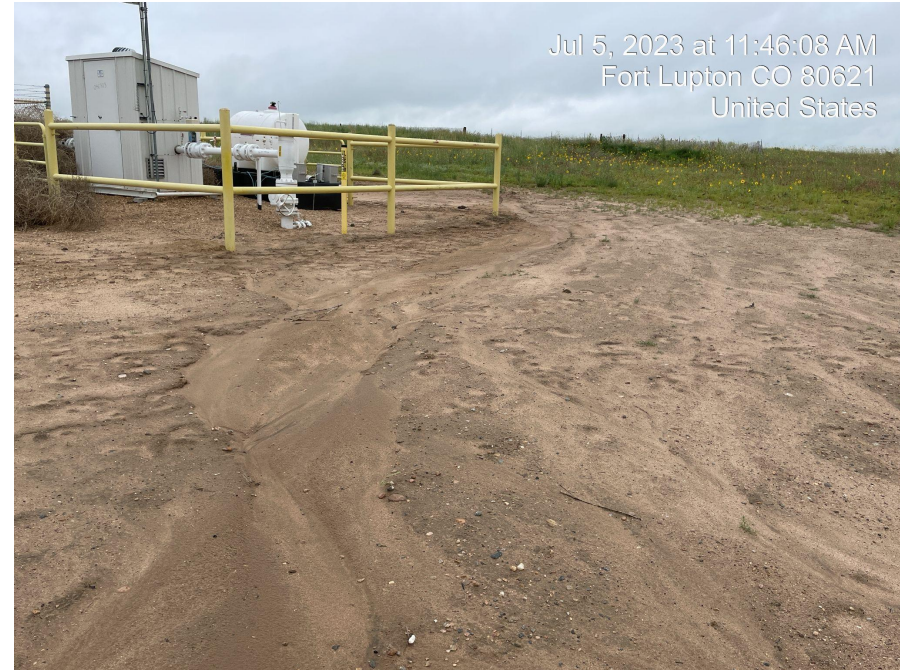
Photo 6. Photo of stormwater erosion on site.
