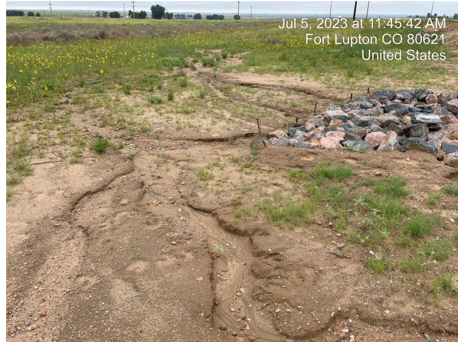
Photo 4. Photo of stormwater erosion bypassing rock rundown.
