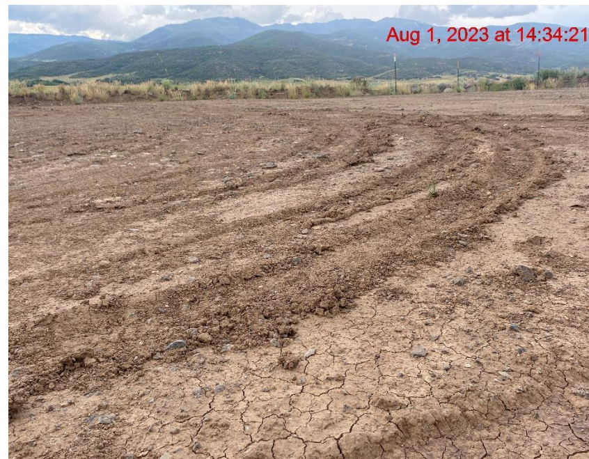
Location Lacks Stabilization – Photo #05323
