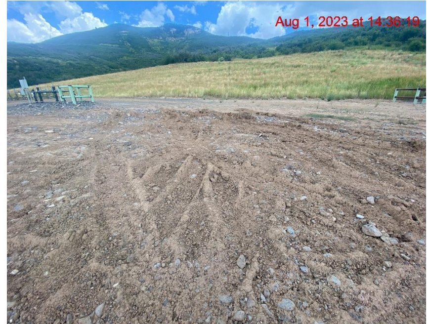
Location Lacks Stabilization – Photo #05328
