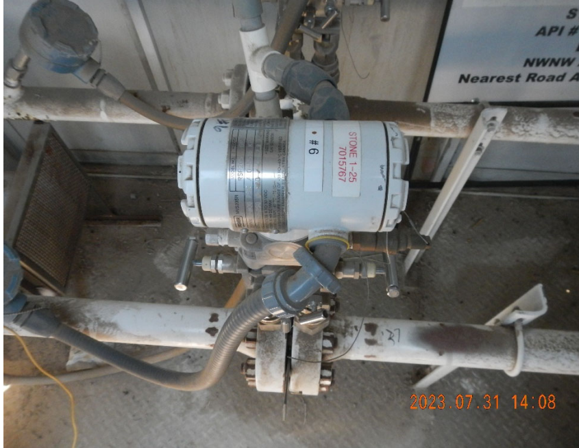
5. Digital Gas Meter inside Meter Shed.
