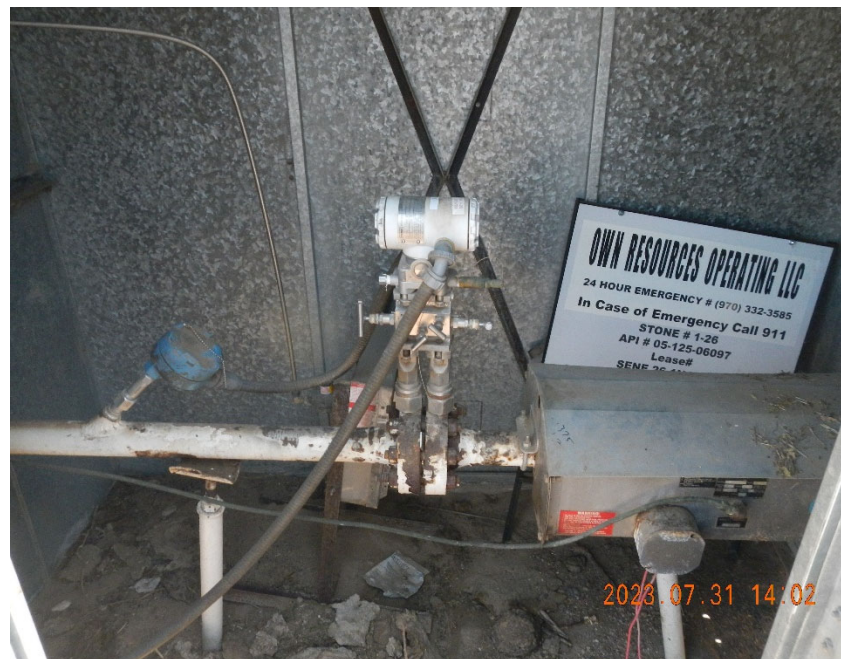
. Digital Gas Meter inside Meter Shed.
