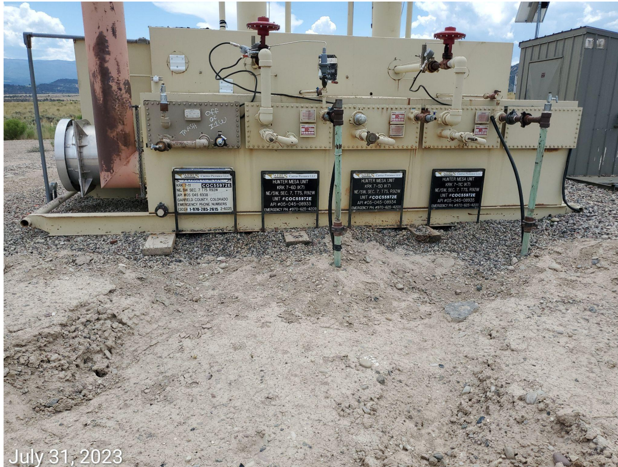
Photo 7: Separator equipment. Flowlines associated with the PA wells appear to have been abandoned/removed.
