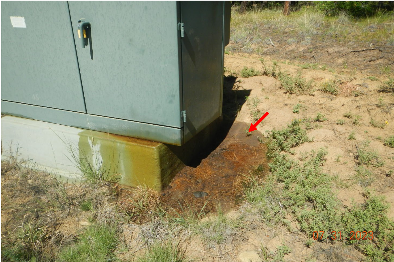
Photo 2. There is oil stained soils at the electric utility that needs to be cleaned up.
