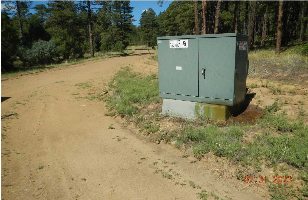
Photo 1. Facing northeast along the access road at Latitude: 37.00784 Longitude: -104.858674. This electric utility is leaking oil that needs to be repaired and cleaned up.
