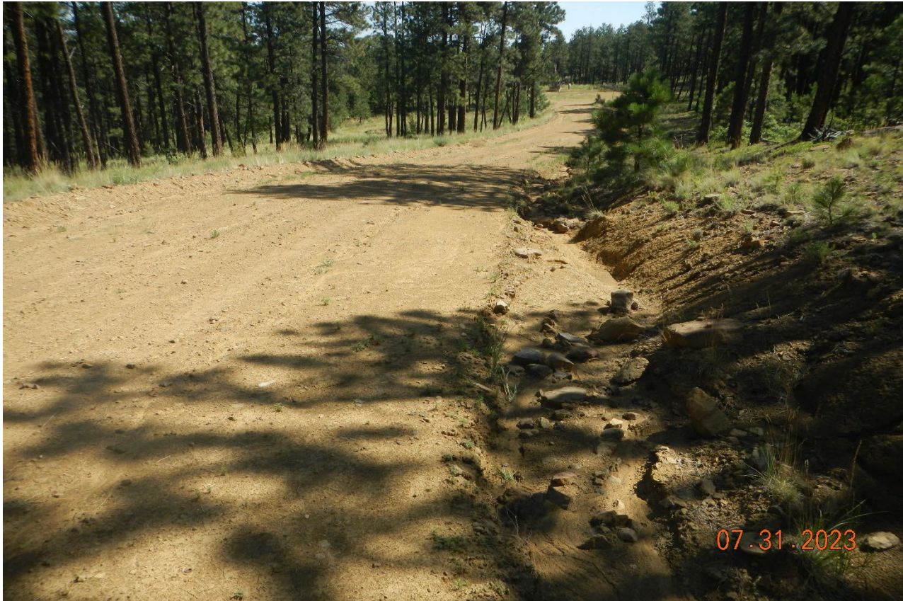
Photo 3. Facing northeast along the access road. There is erosion along the roadside which needs BMP's to control erosion.
