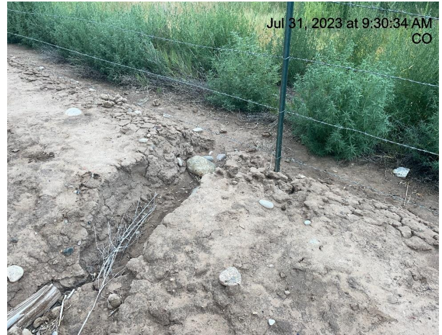
Photo # 4164 Berm needs maintenance - erosion through berm & transport of sediment off location
