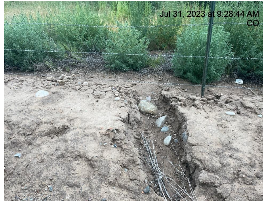
Photo # 4162 Berm needs maintenance - erosion through berm & transport of sediment off location
