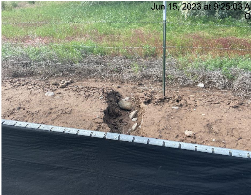
Photo # 502 From inspection 708900775 conducted on 06/15/2023 Berm needs maintenance – erosion through berm & transport of sediment off location
