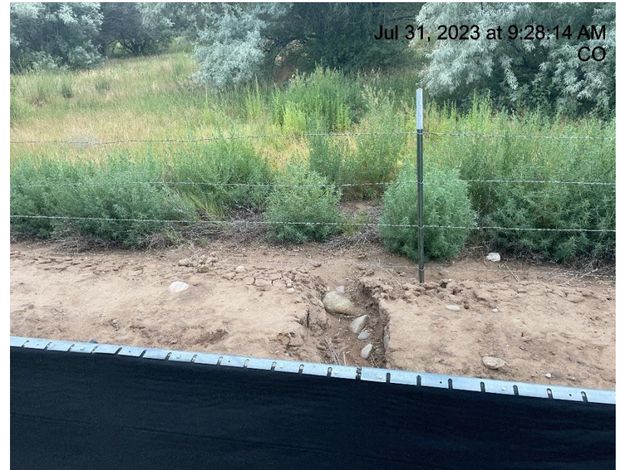
Photo # 4161 Berm needs maintenance - erosion through berm & transport of sediment off location
