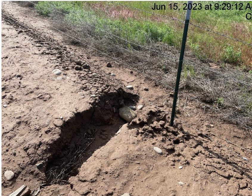
Photo # 510 From inspection 708900775 conducted on 06/15/2023 Berm needs maintenance – erosion through berm & transport of sediment off location
