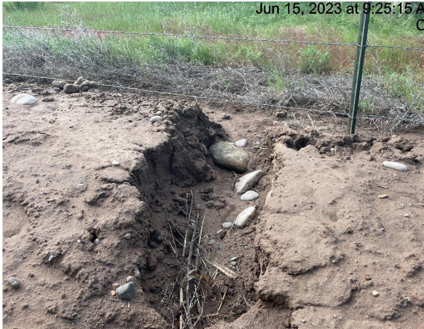
Photo # 503 From inspection 708900775 conducted on 06/15/2023 Berm needs maintenance – erosion through berm & transport of sediment off location
