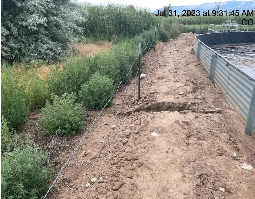
Photo # 4169 Berm needs maintenance – erosion through berm & transport of sediment off location/Failure to minimize erosion & transport of sediment off location
