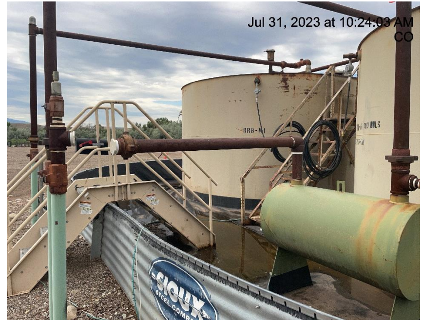
Photo # 4248 ECD line disconnected at tank battery
