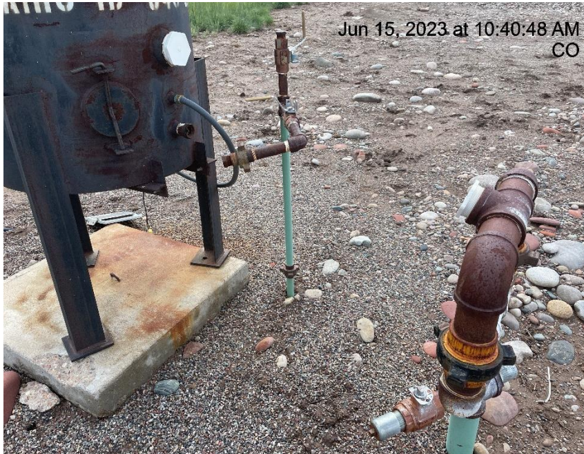
Photo # 595 From inspection 708900778 conducted on 06/15/2023 Unused equipment/ECD is disconnected
