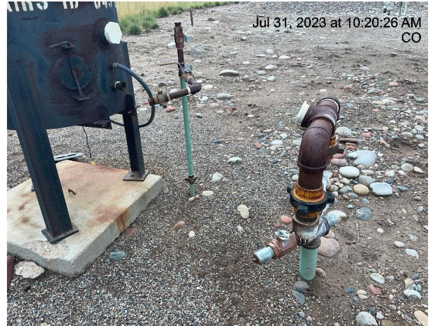
Photo # 4228 Unused equipment/ECD is disconnected
