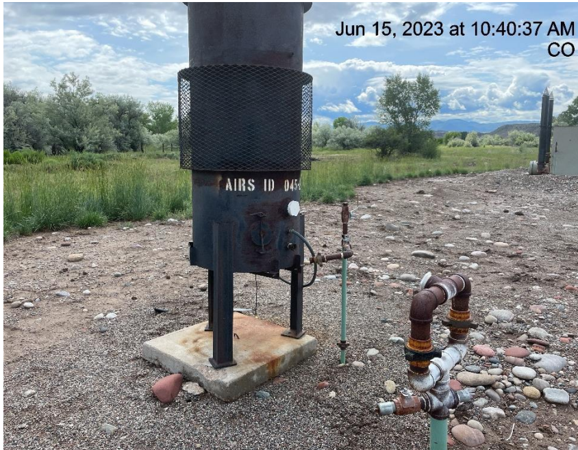
Photo # 594 From inspection 708900778 conducted on 06/15/2023 Unused equipment/ECD is disconnected
