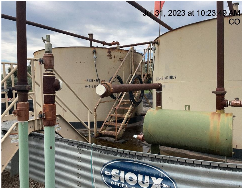
Photo # 4246 ECD line disconnected at tank battery
