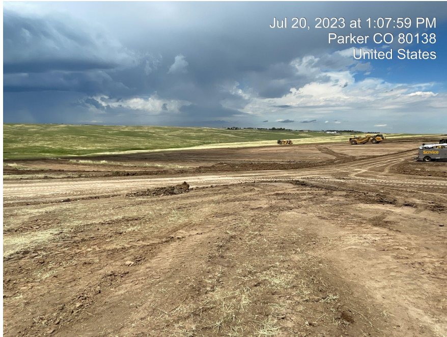
Photo 3. Photo of scraping topsoil.
