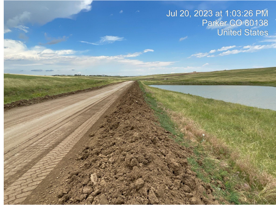
Photo 2. Photo of wind rowed soil on access road, No stormwater BMPs present.
