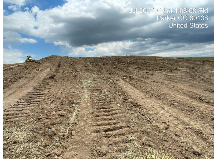
Photo 4. Photo of topsoil stockpile.
