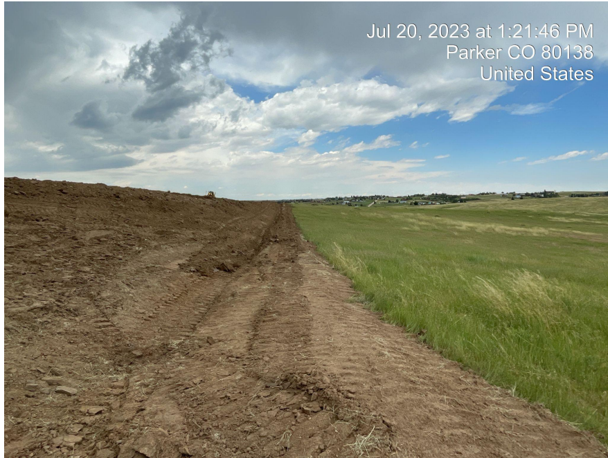
Photo 7. Photo of perimeter ditch on fill slope side.
