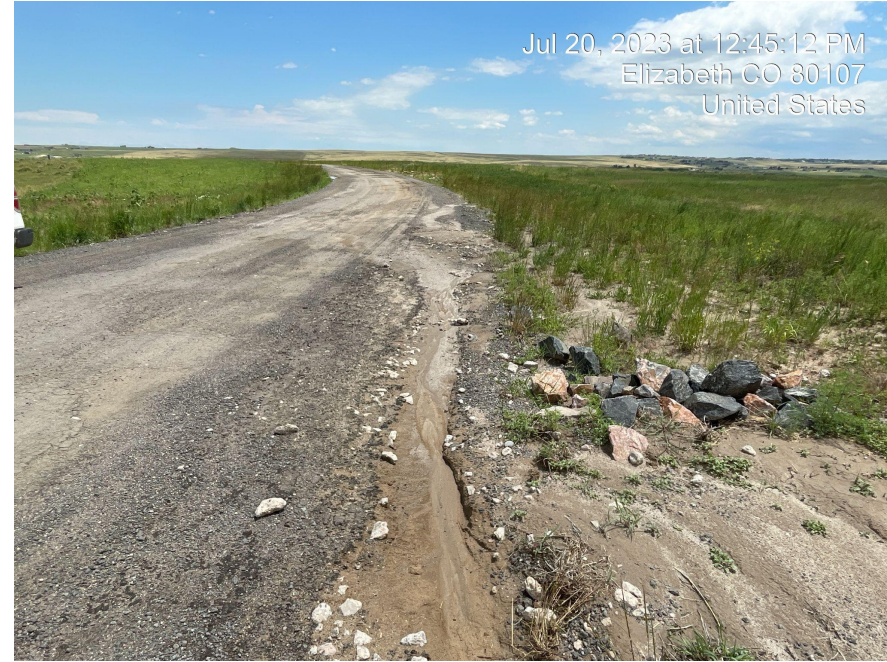
Photo 12. Rock check dam in access road filled with sediment, stormwater has bypassed the BMP.
