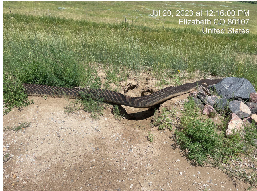
Photo 8. Photo of wattle undermined by stormwater.
