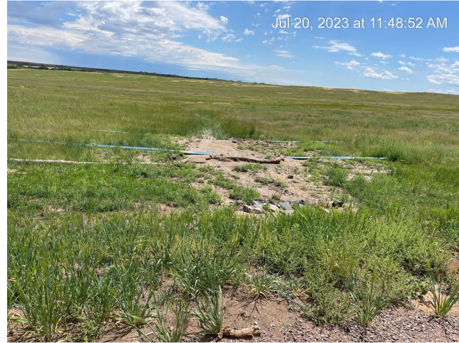
Photo 10. Photo of pipe parallel to access road capturing sediment carried off site by stormwater.
