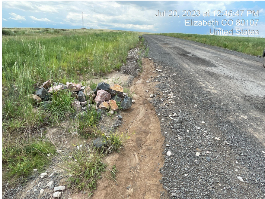
Photo 9. Photo of stormwater by passing rock check dam in access road.
