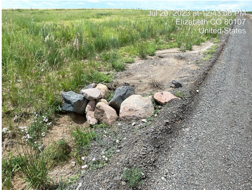
Photo 11. Photo of rock check dam in access road that has been tunnelled under by stormwater.
