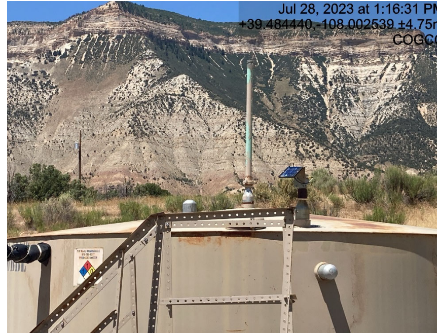
Line on tank open to atmosphere
