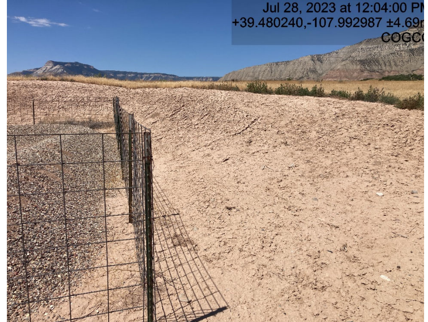
Lack of stabilization and erosion
