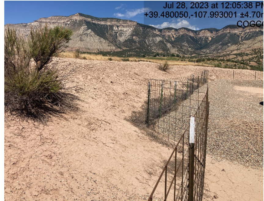
Cut slope lacks stabilization and Weeds have turned in to debris
