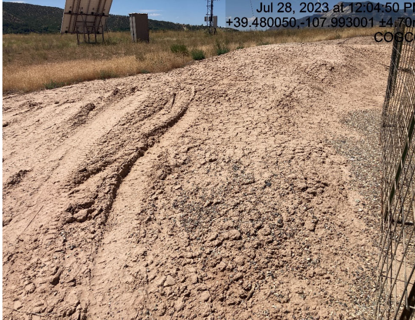
Lack of stabilization and erosion
