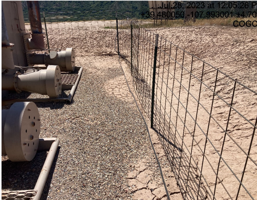
Lack of stabilization, erosion and sediment migration encroaching on production equipment
