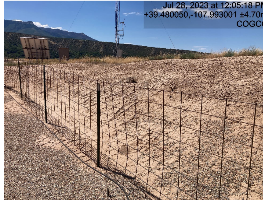
Lack of stabilization, erosion and sediment migration encroaching on production equipment
