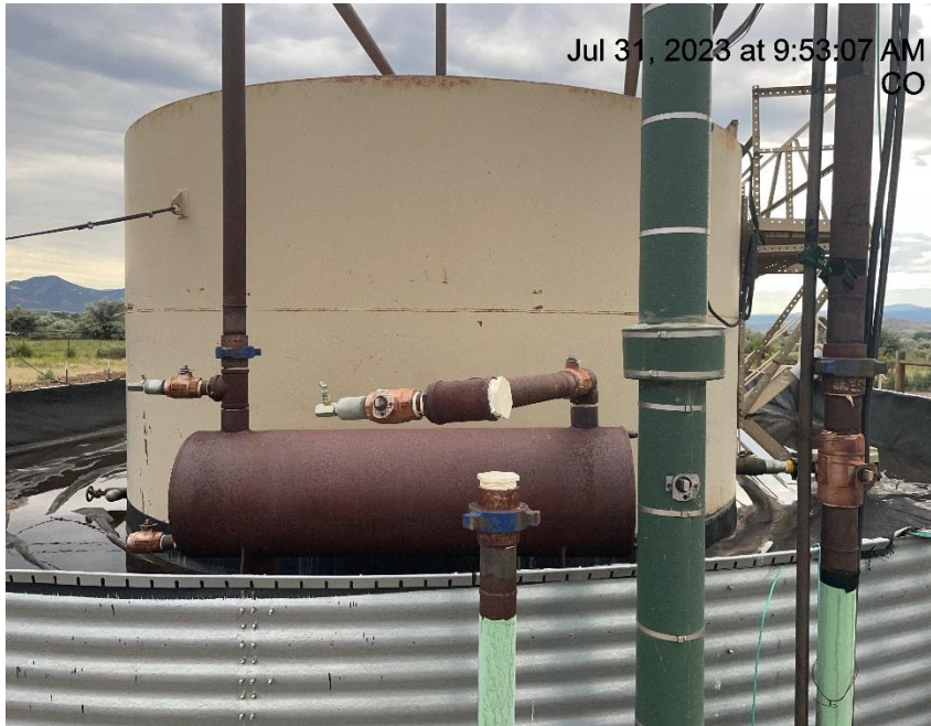
Photo # 4188 ECD line disconnected at tank battery
