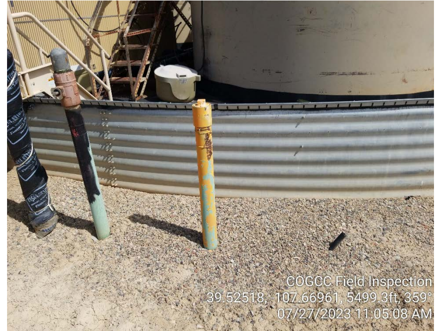
Photo #4 – Marked, unused flowline riser located on south end of tank battery.
