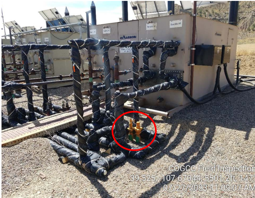
Photo #9 – Additional marked, unused flowline risers located at separator for Burckle A8 well (circled in red).
