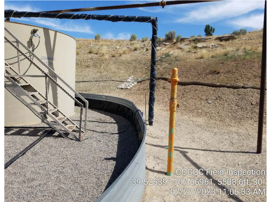
Photo #6 – Marked, unused flowline riser located on east end of northern tank battery.
