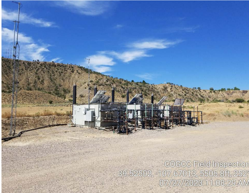
Photo #7 – Horizontal heated separators located on south end of tank battery.
