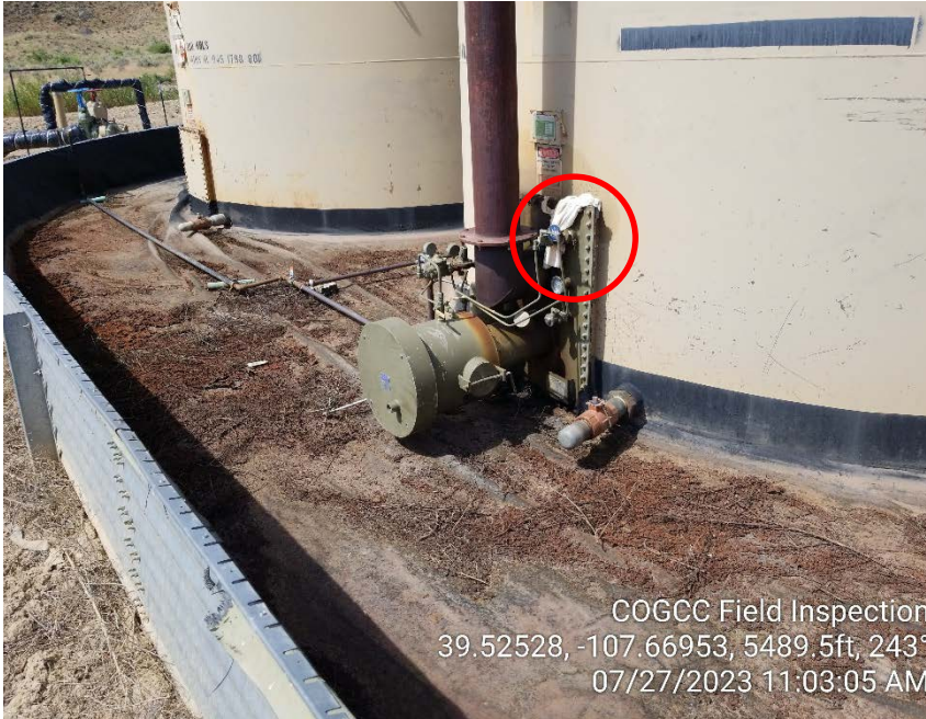
Photo #3 – Localized accumulation of vegetable debris at tank heater. Note red circle documents presence of a rag at the manhole cover, by the heater.
