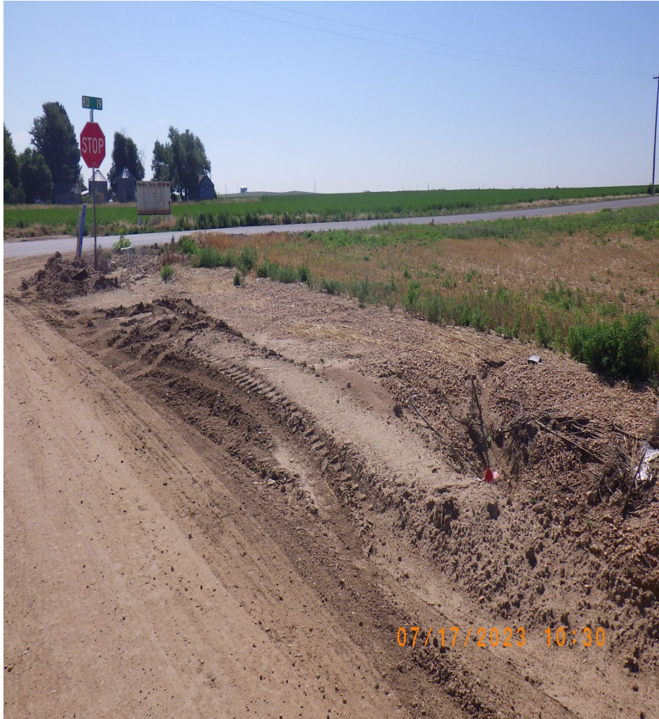
Photo 6. Photos of the tank battery access point and culvert. Photo shows that the operator failed to reclaim the access point and remove culverts.
