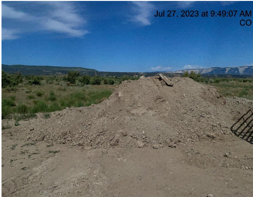
Photo # 3892 Insufficient BMP's for stockpiled soils on location
