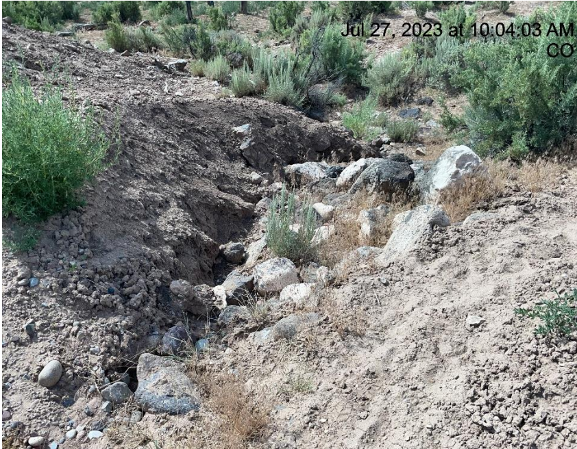
Photo # 3916 BMP needs maintenance (located at 1 st switchback on lease road)
