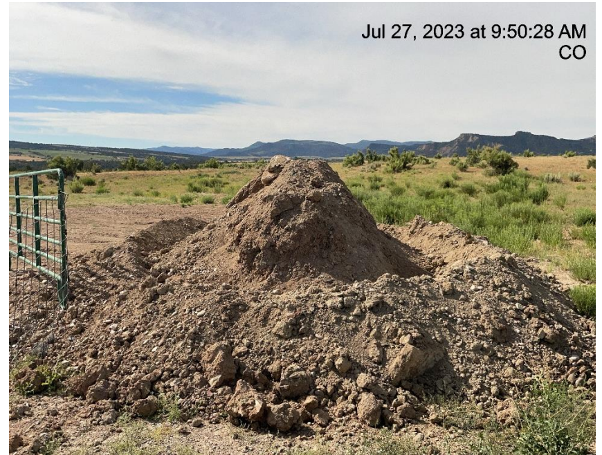
Photo # 3897 Insufficient BMP's for stockpiled soils on location
