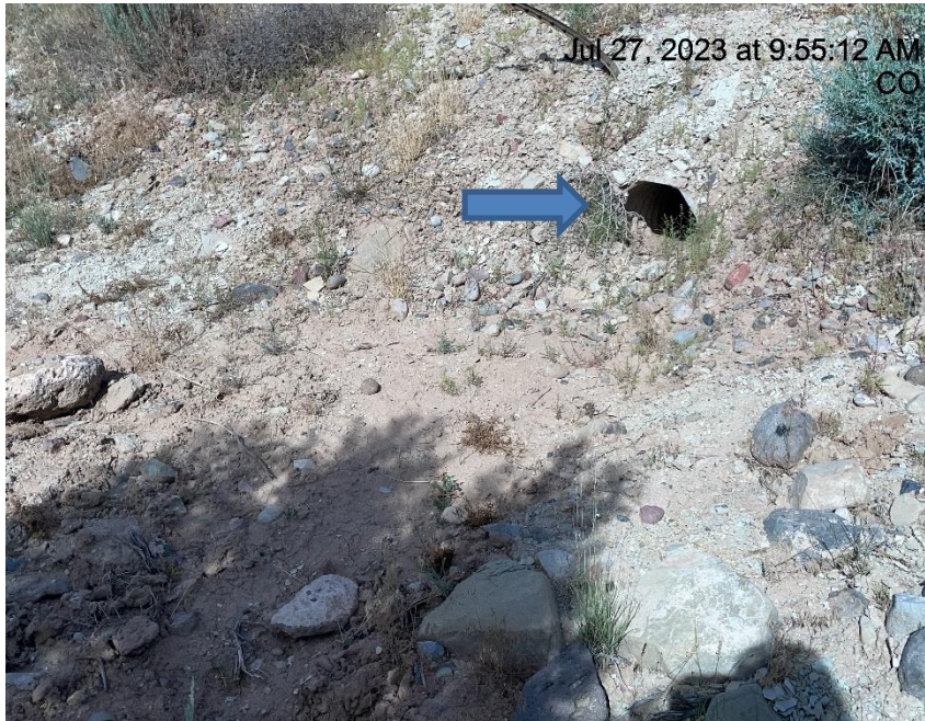
Photo # 3901 Culvert needs maintenance/insufficient BMP's (Culvert approximately 1/10 th of a mile from location on lease road near wattles on lease road)
