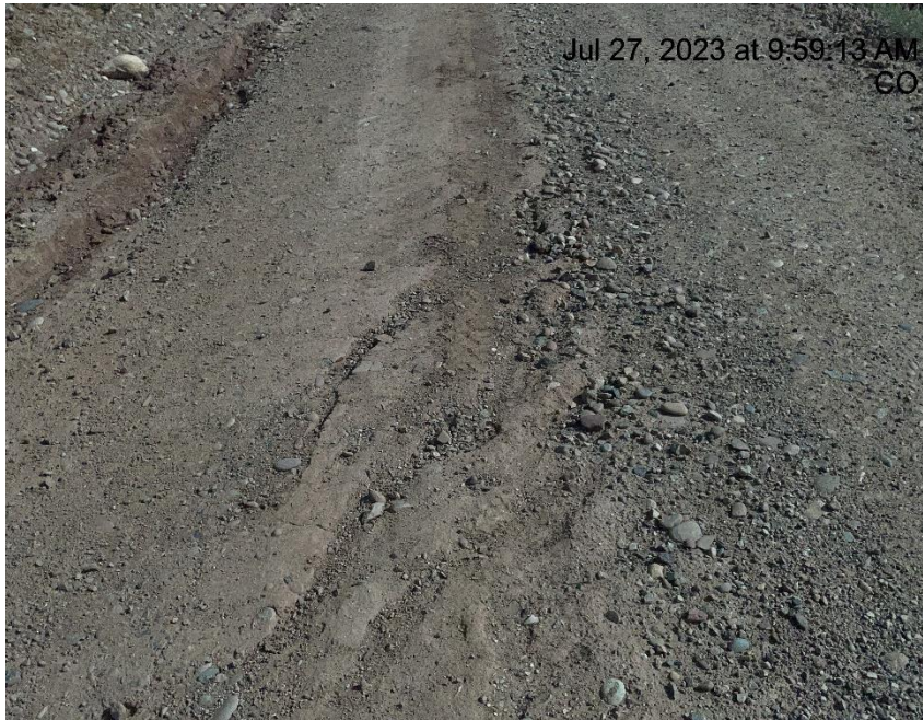
Photo # 3907 Erosion & transport of sediment on lease road (after 1 st switchback on lease road)
