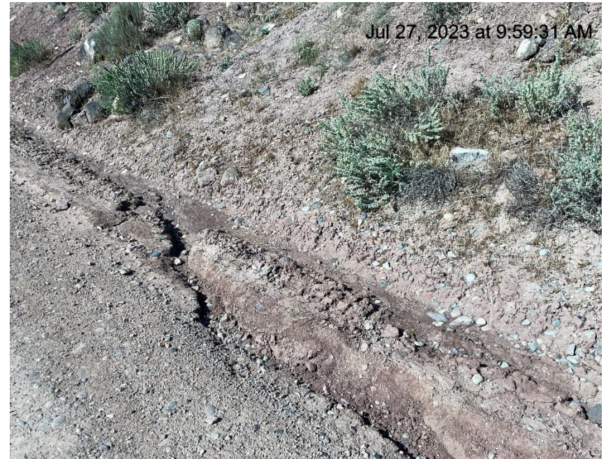
Photo # 3908 Erosion & transport of sediment on lease road
