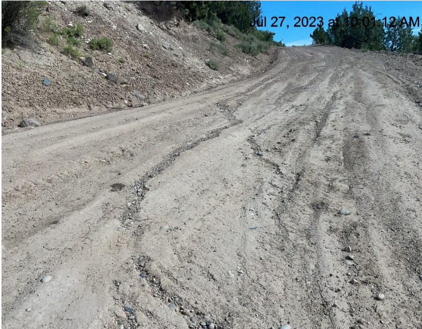
Photo # 3910 Erosion & transport of sediment on lease road (just after 1 st switchback on lease road)
