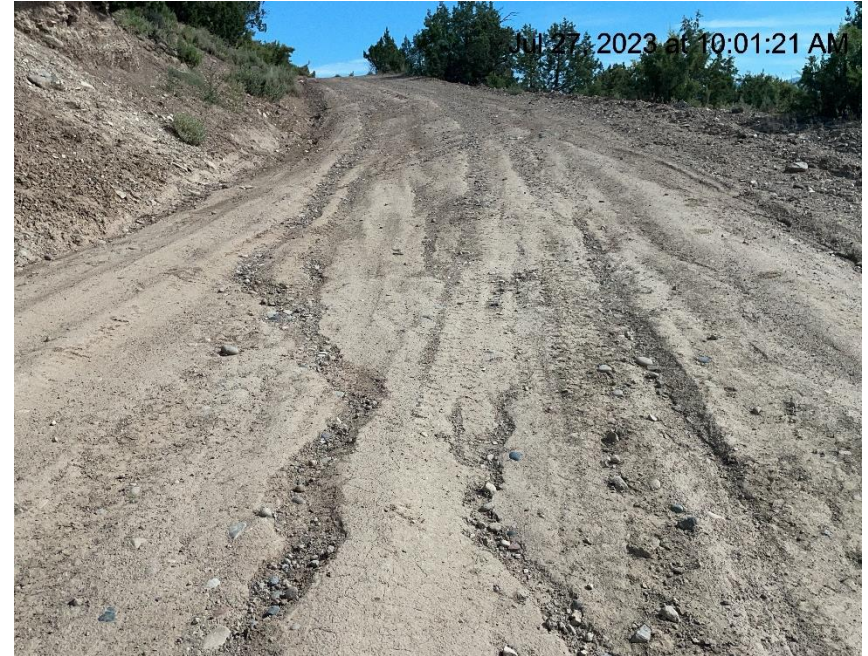
Photo # 3911 Erosion & transport of sediment on lease road (just after 1 st switchback on lease road)
