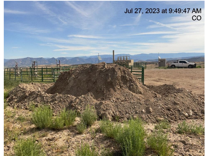
Photo # 3895 Insufficient BMP's for stockpiled soils on location
