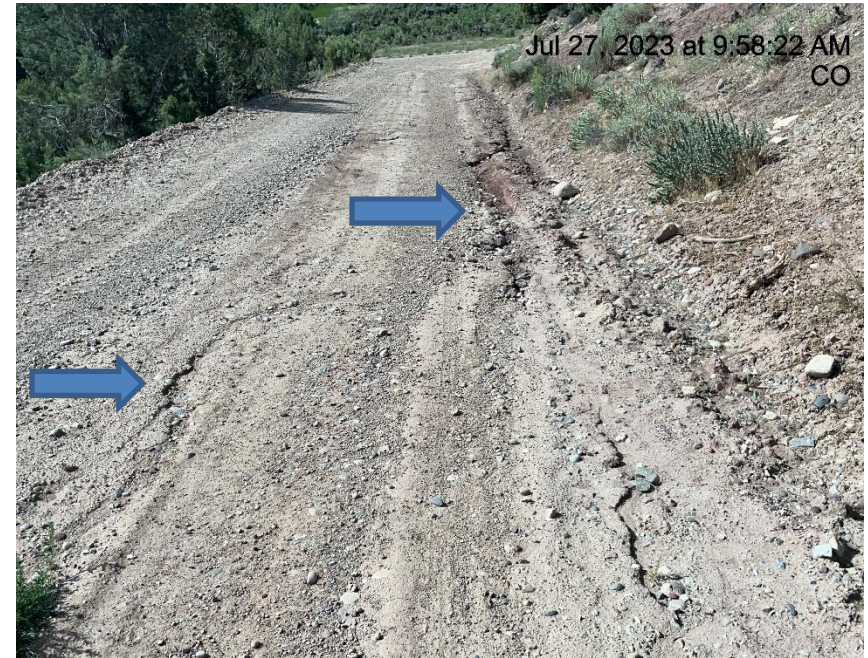
Photo # 3903 Erosion & transport of sediment on lease road (approximately 30-40 yards after 1st switchback on lease road)
