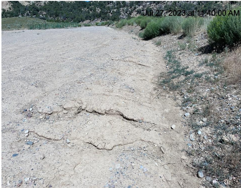
Photo # 4041 Rill erosion & transport of sediment (N/NE area of pad)
