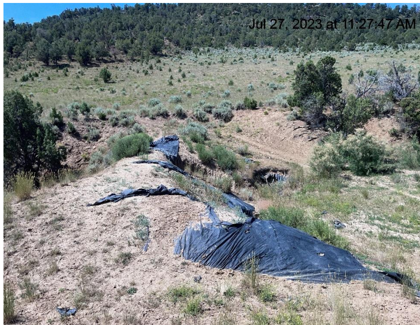
Photo # 4010 Geotextile/liner & erosion observed approximately 25-35 yards S/SW of location
