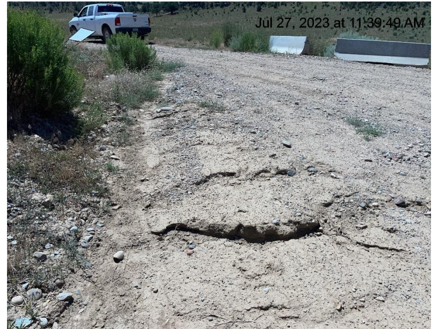
Photo # 4040 Rill erosion & transport of sediment (N/NE area of pad)
