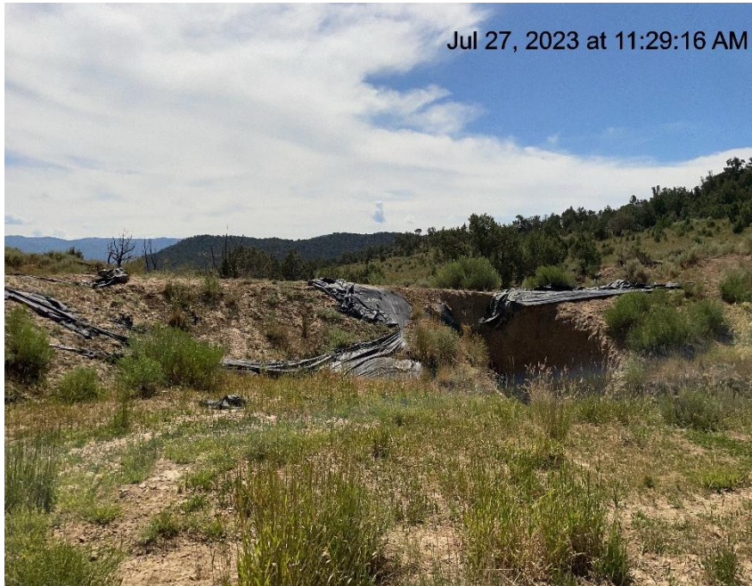
Photo # 4014 Geotextile/liner & erosion observed approximately 25-35 yards S/SW of location
