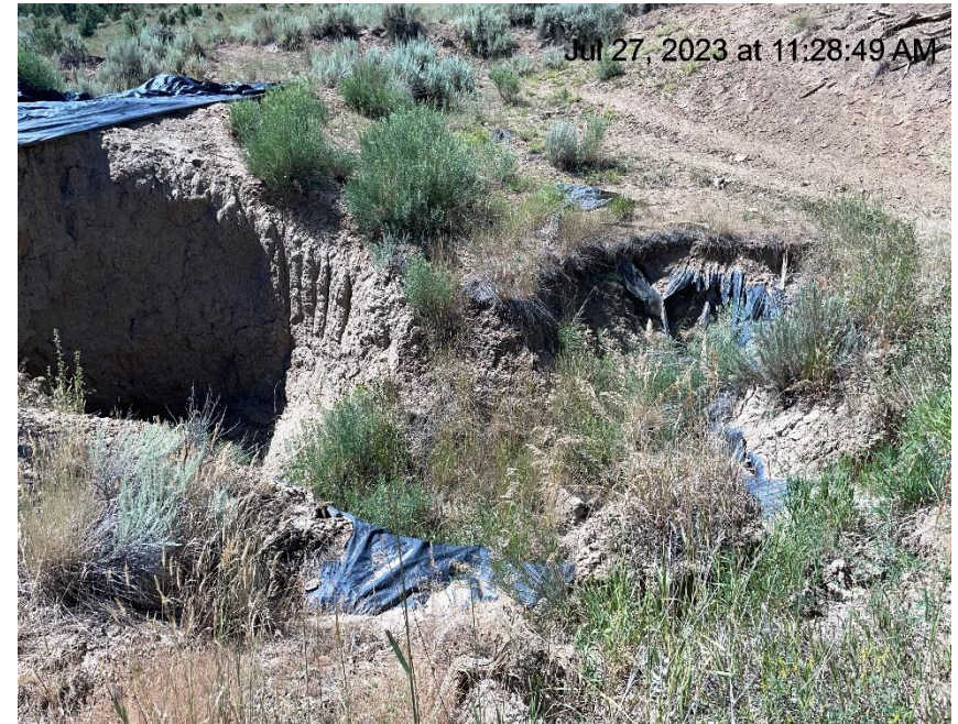
Photo # 4013 Geotextile/liner & erosion observed approximately 25-35 yards S/SW of location
