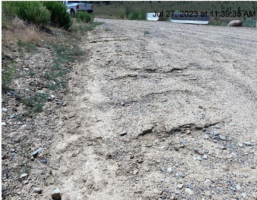
Photo # 4038 Rill erosion & transport of sediment (N/NE area of pad)
