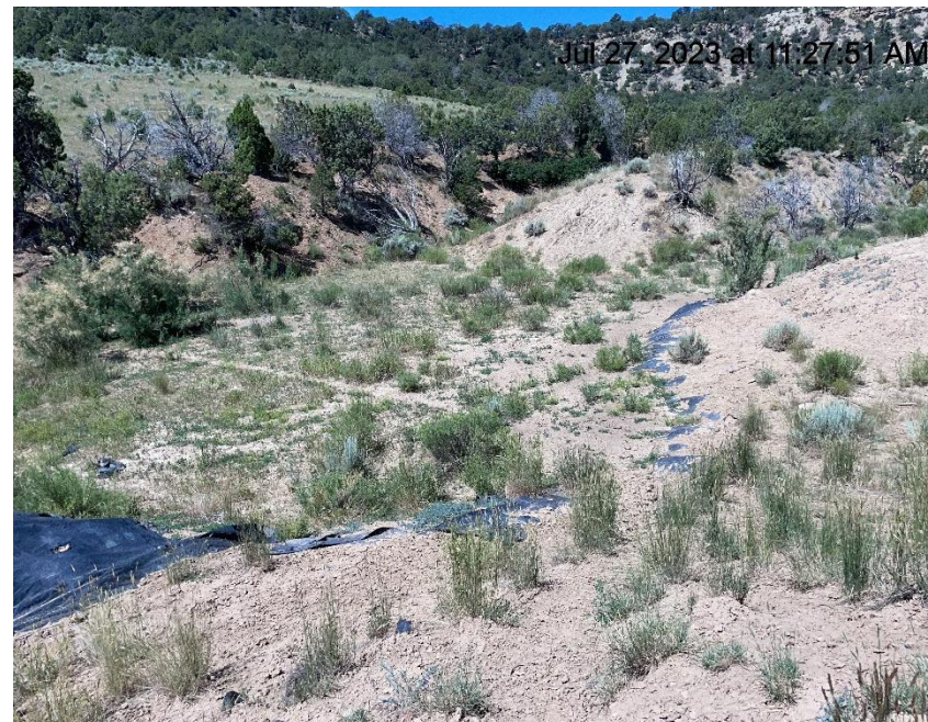
Photo # 4011 Geotextile/liner & erosion observed approximately 25-35 yards S/SW of location
