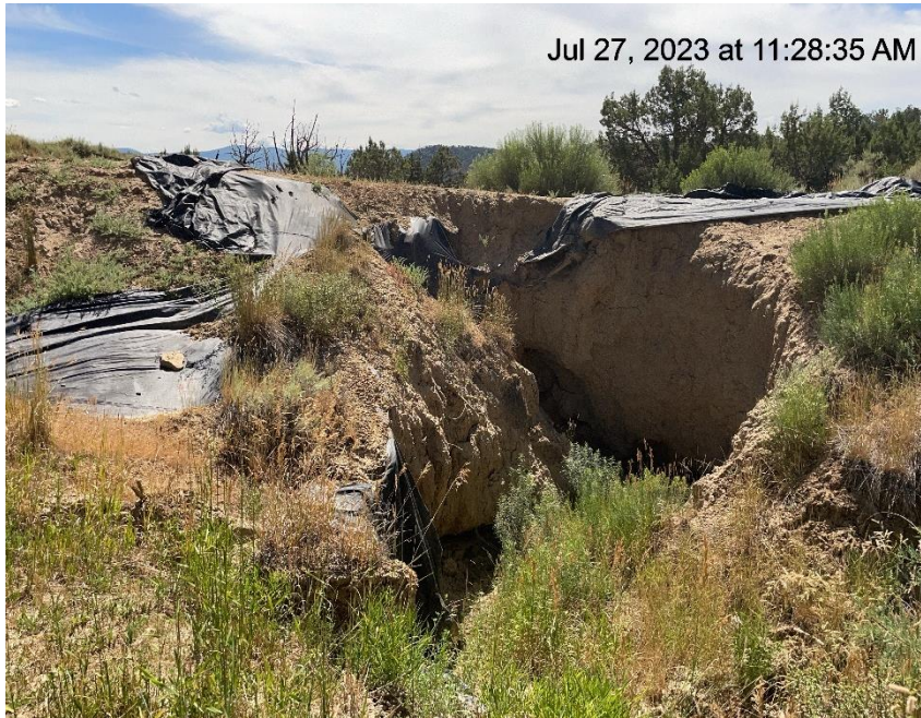
Photo # 4012 Geotextile/liner & erosion observed approximately 25-35 yards S/SW of location
