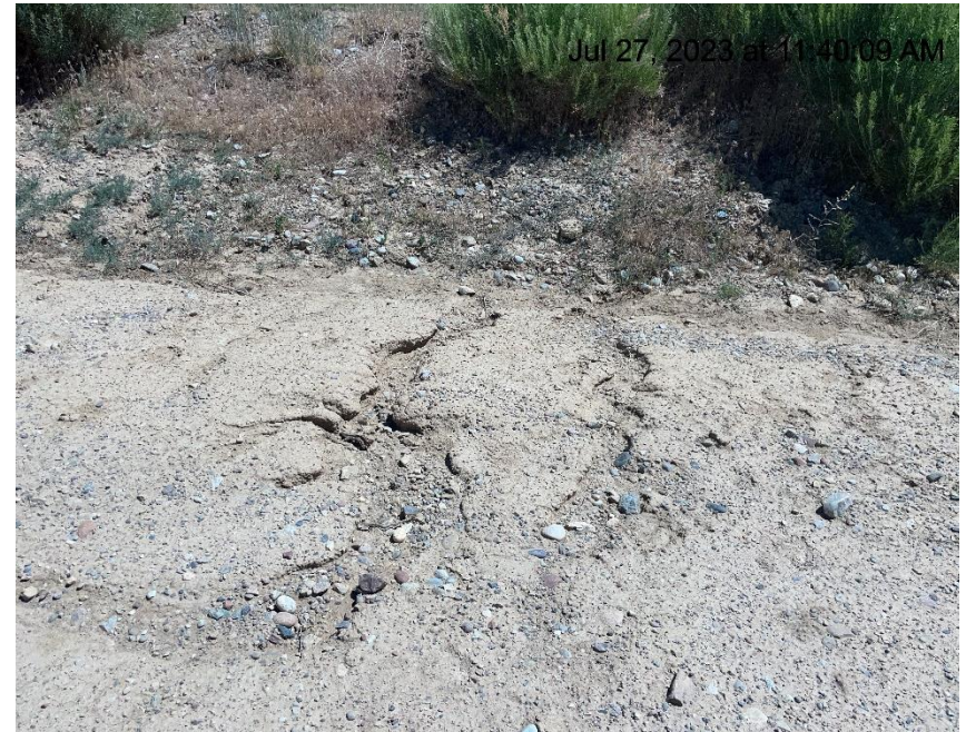
Photo # 4042 Rill erosion & transport of sediment (N/NE area of pad)
