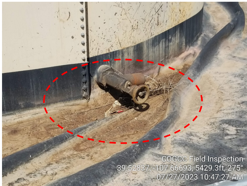
Photo #5 - Localized accumulation of oily waste on tank valve (2).
