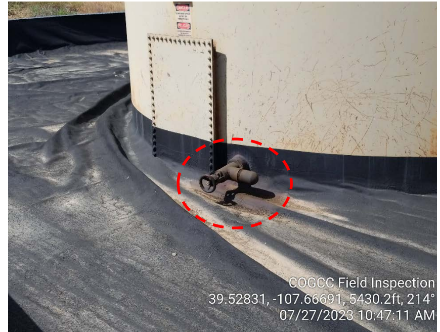
Photo #4 – Localized accumulation of oily waste on tank valve (1).
