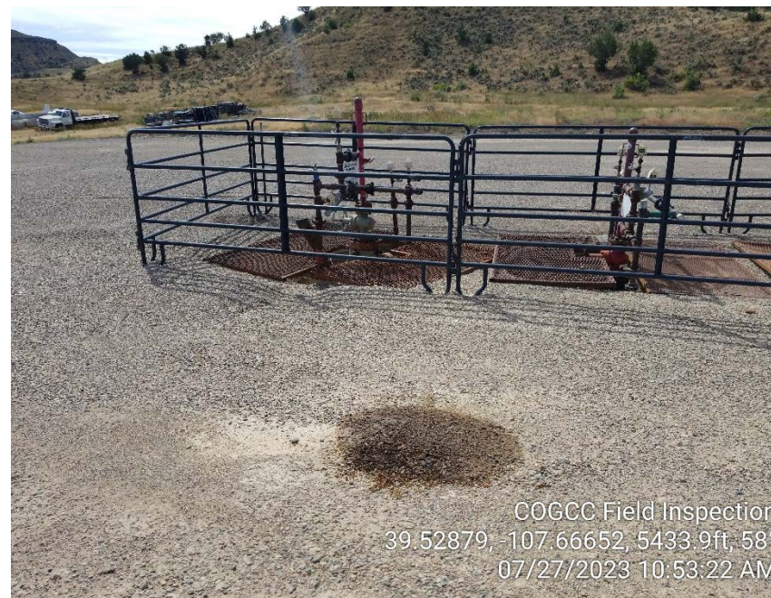
Photo #10 – Localized accumulation of oily waste located northeast of wells.
