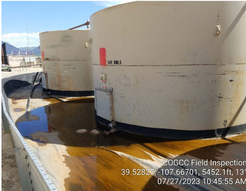
Photo #3 – Fluids observed in tank battery secondary containment area.
