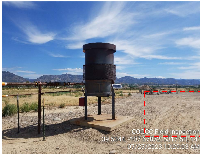
Photo #5 – Emissions Control Device. Note, red box denotes stabilization and compaction issues remaining from previous inspection (doc #707800316).
