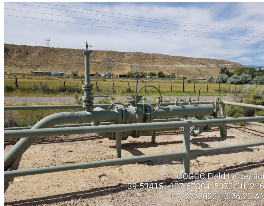
Photo #2 – Pipeline manifold in SW corner of pad.
