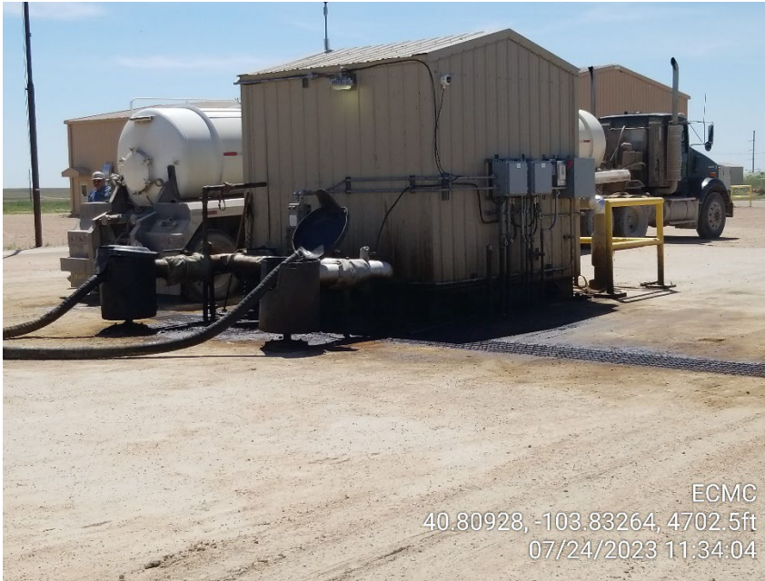
Photo 5 – East Truck Loadout – Stained Soil and Oily Waste
