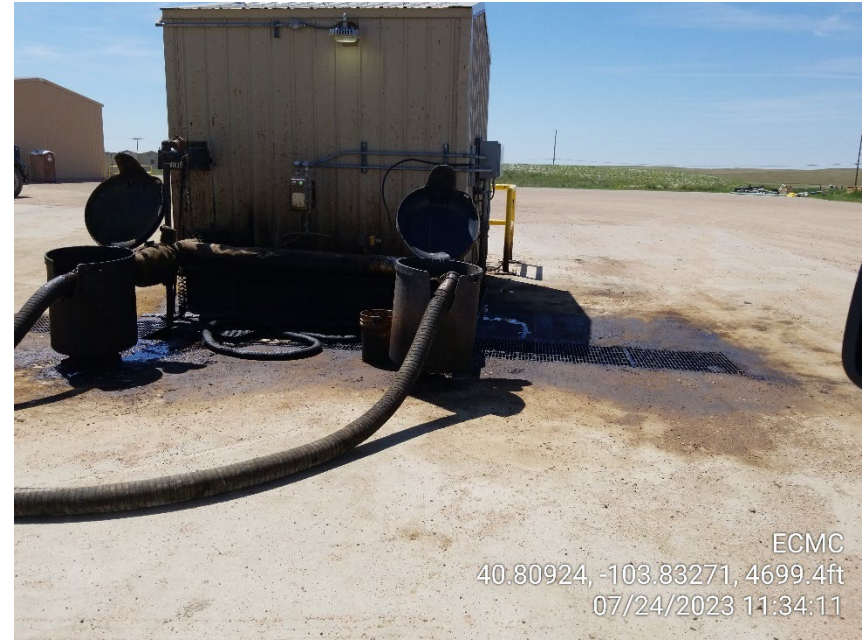
Photo 6 – West Truck Loadout – Stained Soil and Oily Waste
