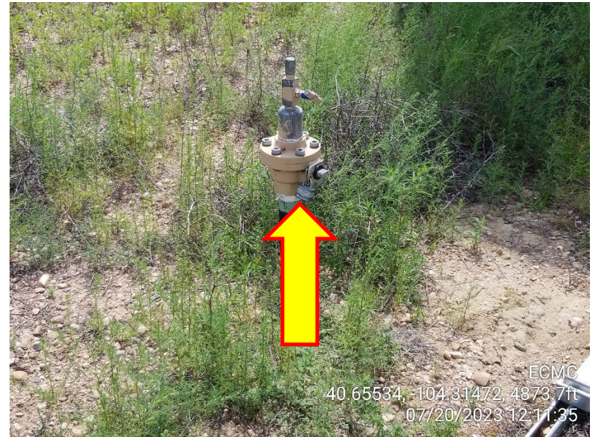
Photo 4 – Riser has been Locked Out
