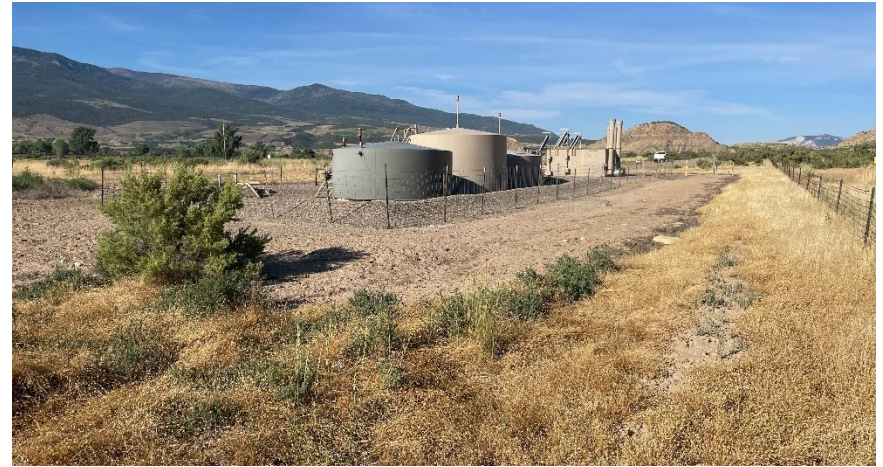
North East corner of location.
