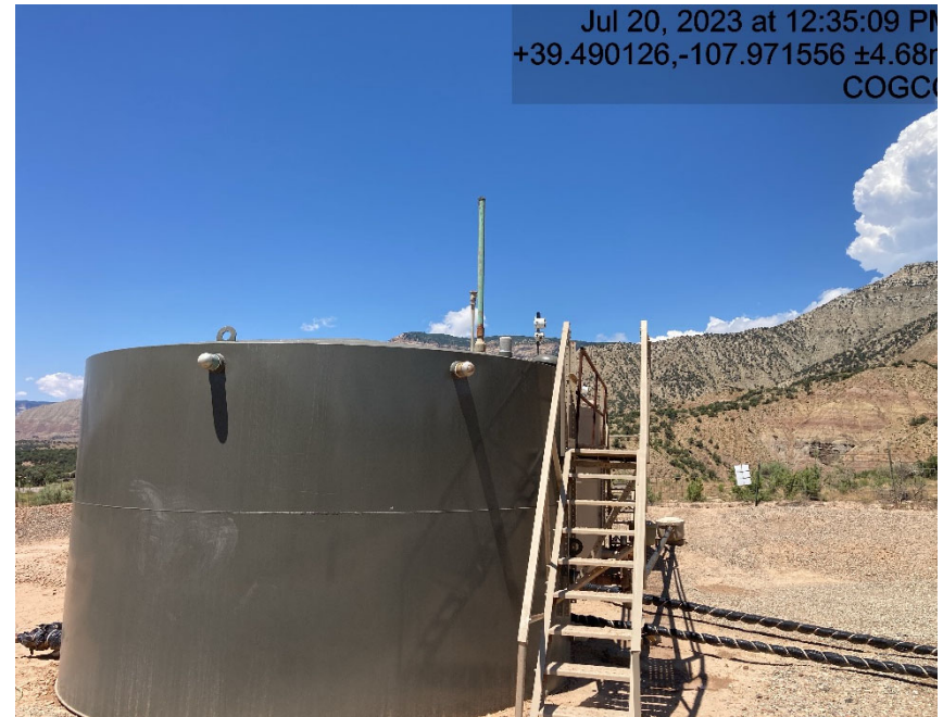
Tank has line on top open to atmosphere
