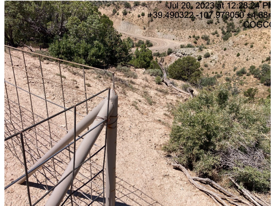
Lack of BMP's on edge of location to prevent sediment migration
