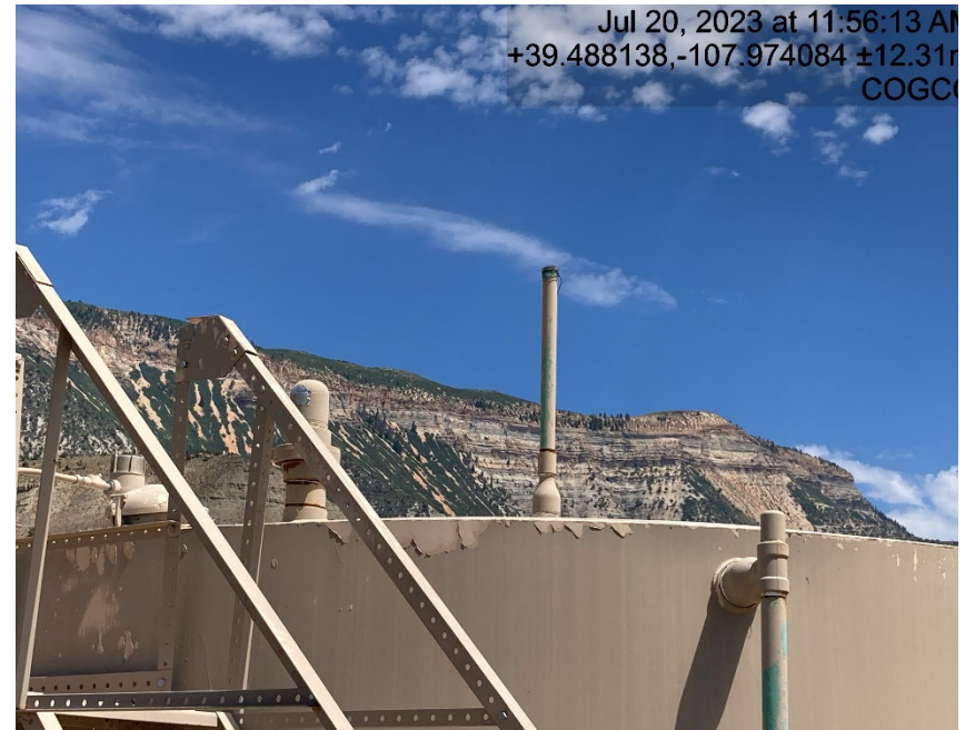
Line on tank open to atmosphere
