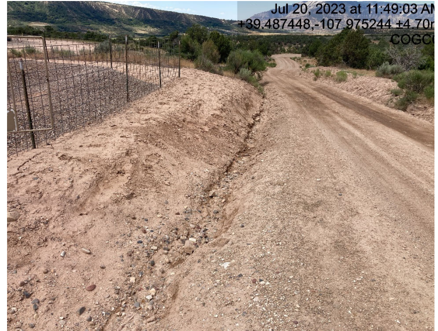
Ditch on side of location lacks erosion control
