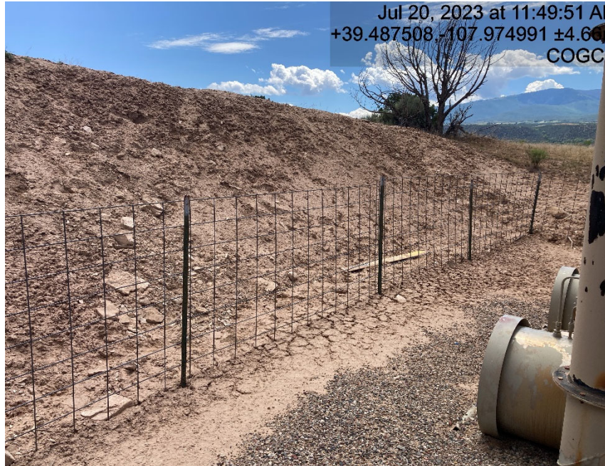
Cut slope lacks stabilization and migrating onto location encroaching on production equipment
