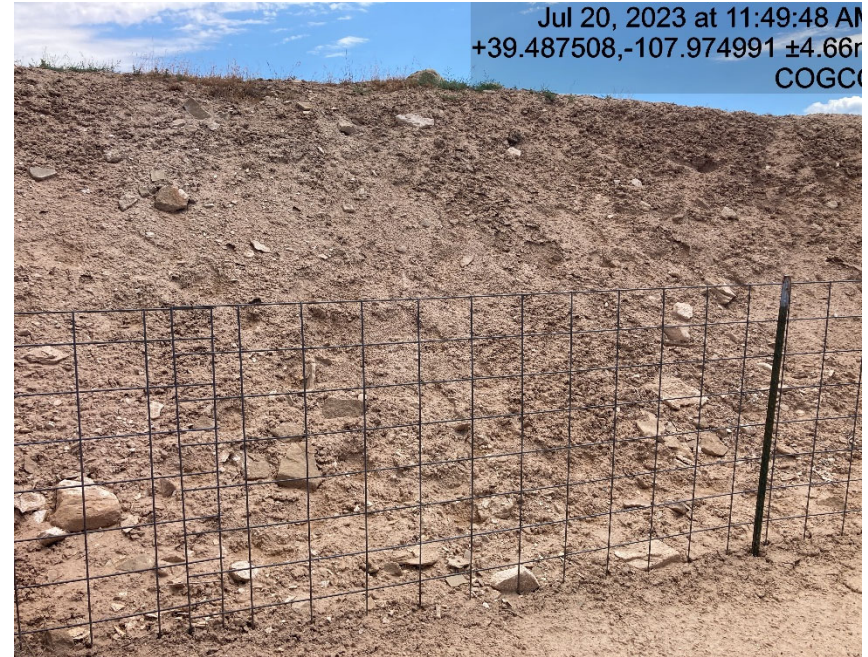
Cut slope lacks stabilization and migrating onto location encroaching on production equipment
