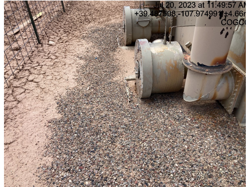
Sediment migrated over skid of production equipment
