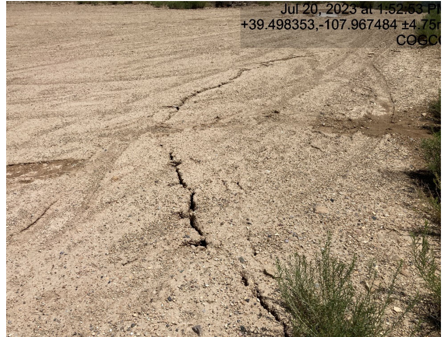
Ground has crack in it to edge of location, sign of lack of stabilization
