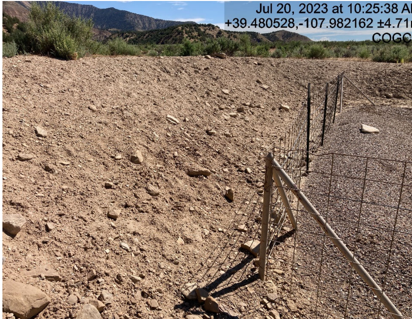
Lack of stabilization on cut slope
