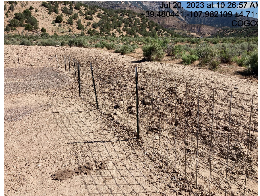
Lack of stabilization on cut slope
