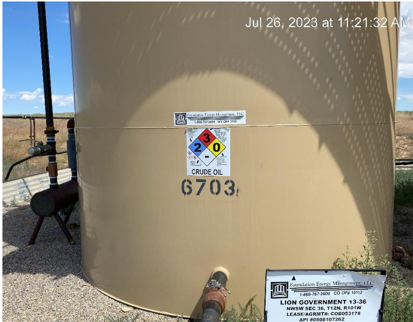
Missing tank capacity
