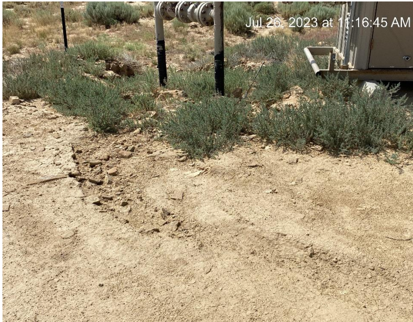
Erosion and sediment migration from location
