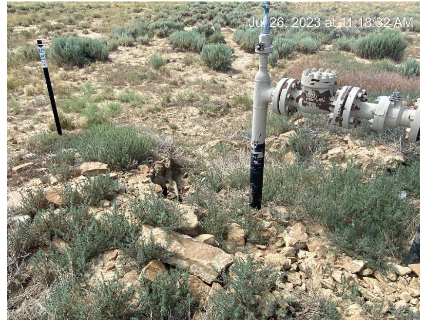
Erosion and sediment migration from location
