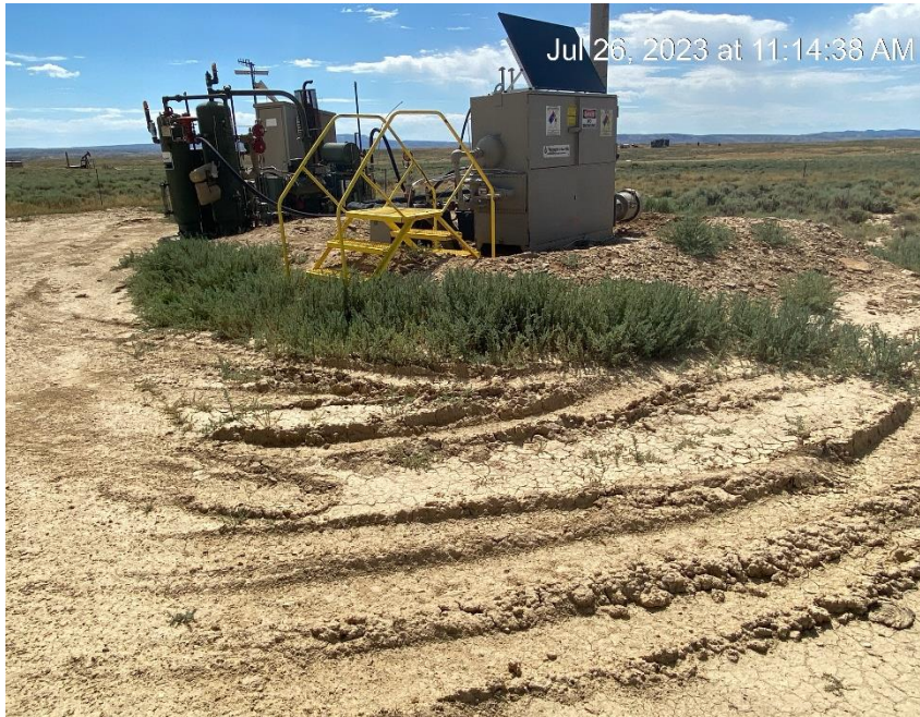
Lack of stabilization. Weeds. Vehicle tracking.
