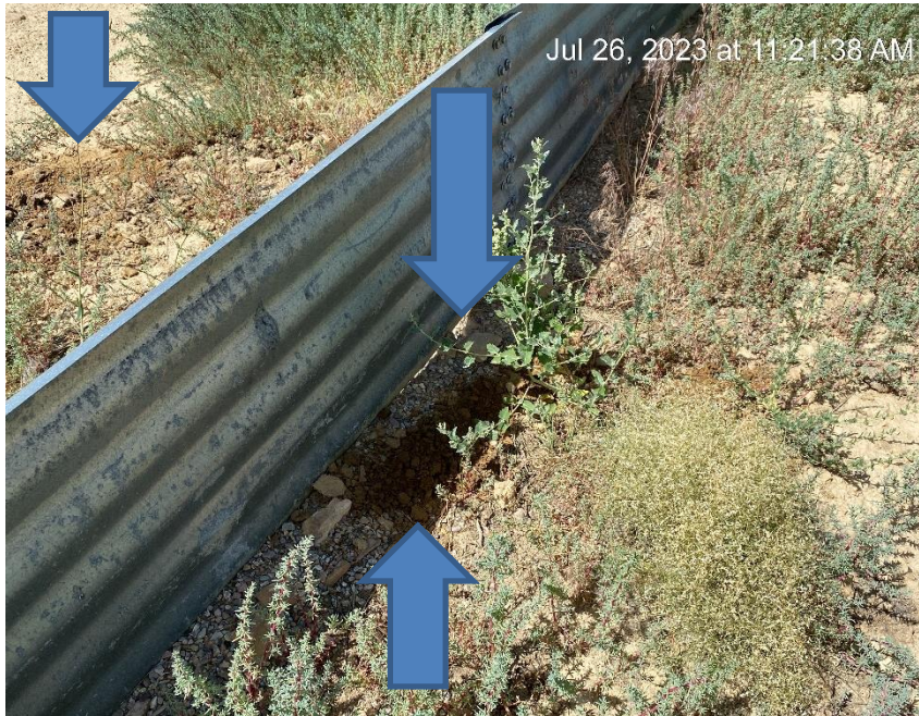
Stained soil, weeds and opening in metal berm
