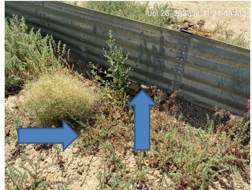
Stained soil, weeds and opening in metal berm
