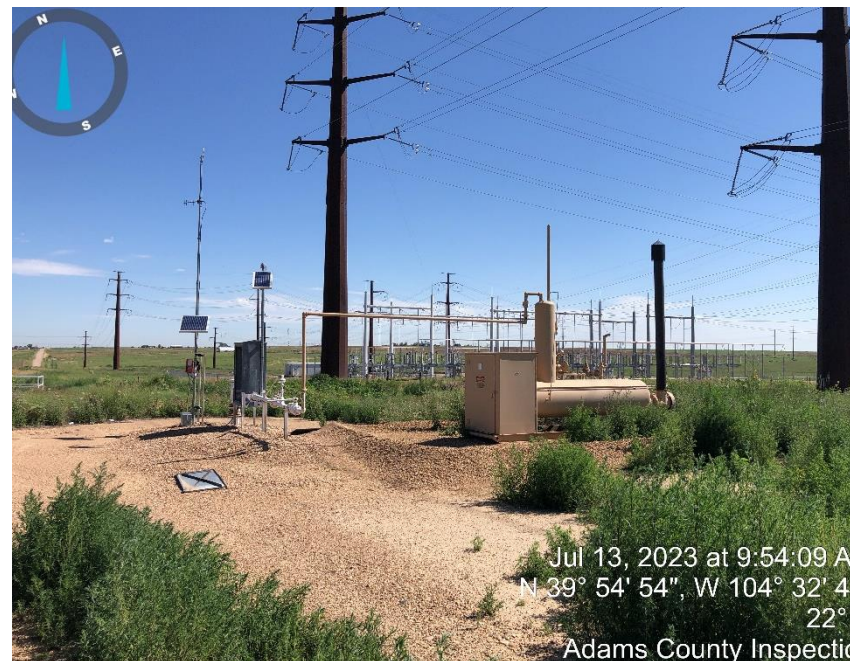
Photo# 2 Separator & meter.
