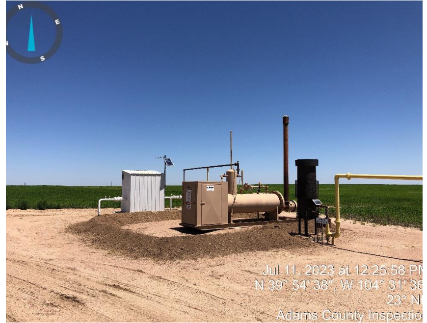
Photo# 2 Separator and meter run
